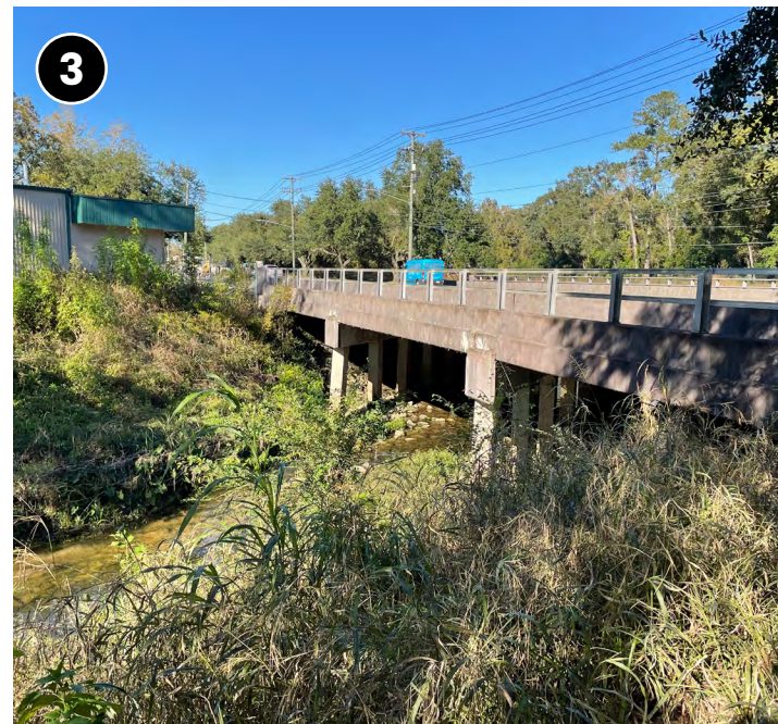
View under Springhill Rd bridge facing north
