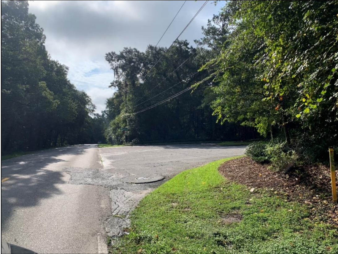
Intersection of Millers Bridge Road and Maclay Road
