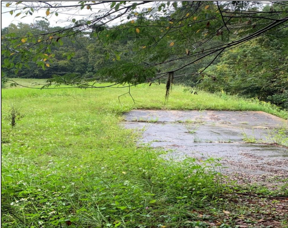
Existing Detention Pond Concrete Spillway
