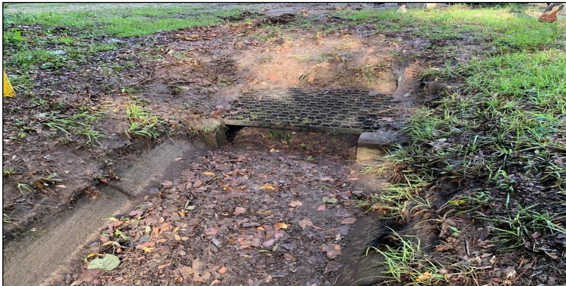
Existing Drainage Structure
