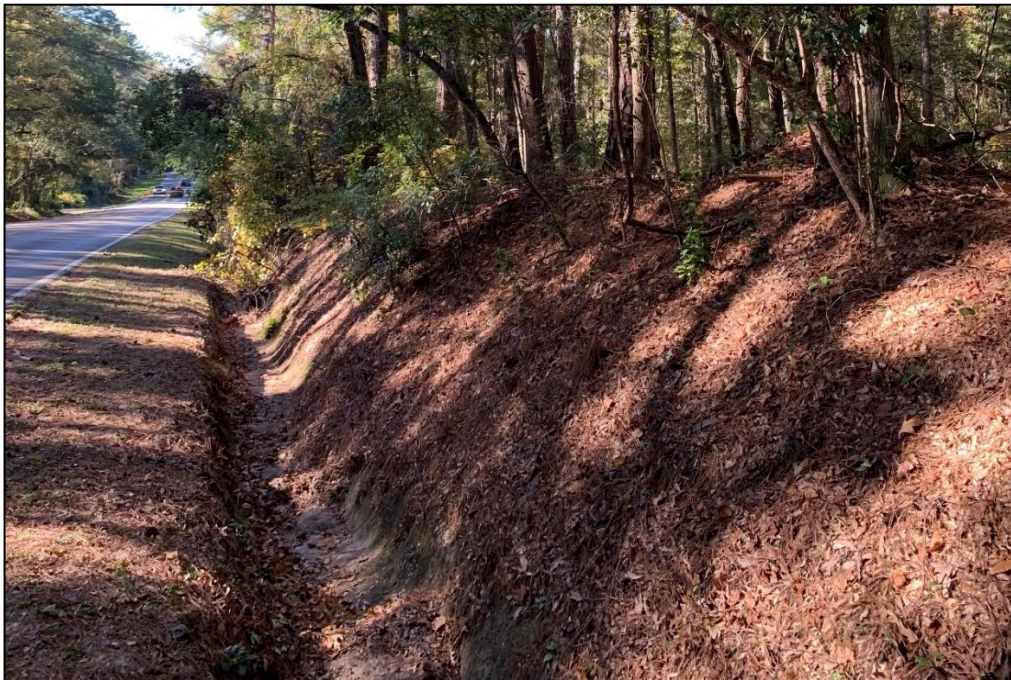
North Side Limited Space Area
