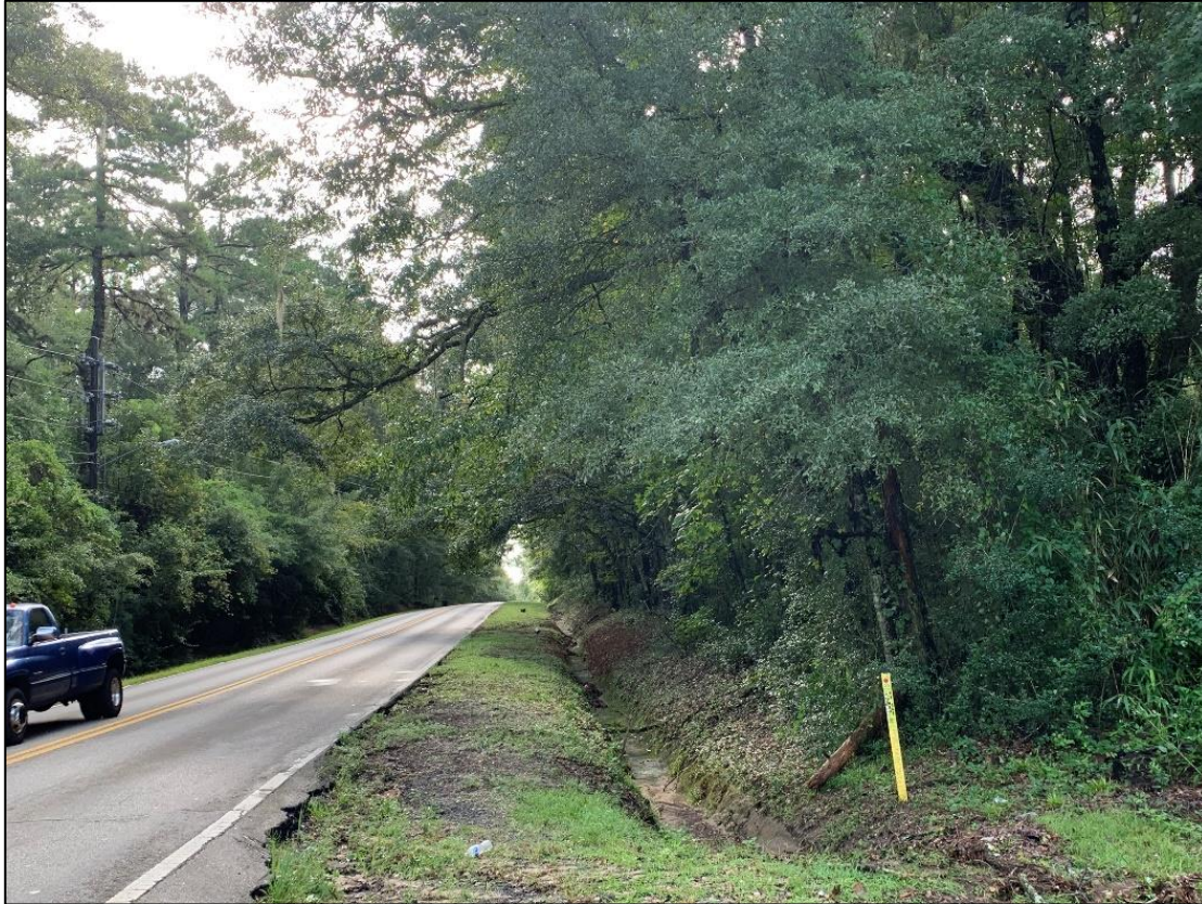
South Side Concrete Ditch Pavement
