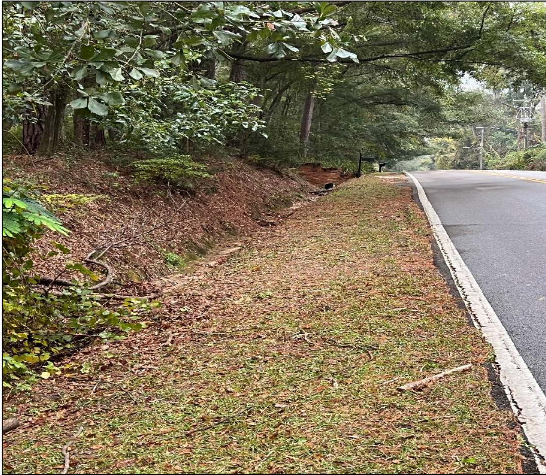
North side Concrete Ditch Pavement
