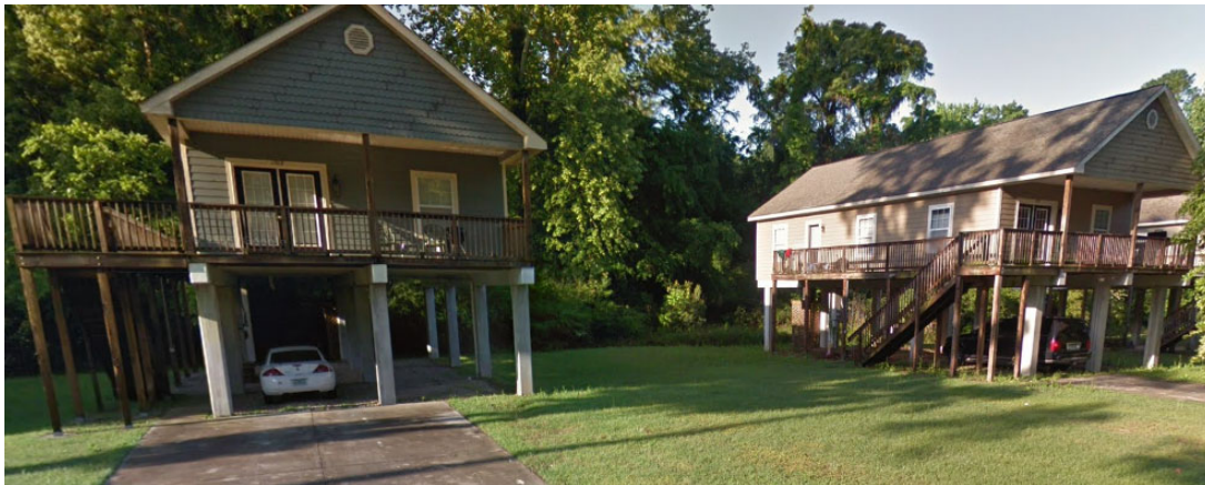
Figure 13 Flood Protection Example – Elevated Homes Along McPhearson Drive
