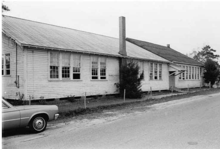
Figure 20. Barrow Hill School Building, side view (November 11, 1965). (State Archives of Florida, Florida Memory).
