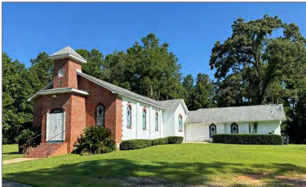
Figure A-1. Testerina Primitive Baptist Church, located at 5520 Miccosukee Road, facing northwest.
