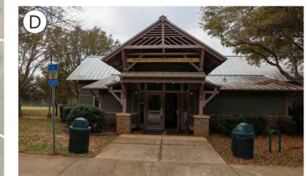
Concession / Community Room / Restroom Building
