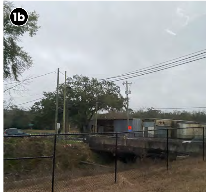
View of Kissimmee Street bridge from the north
