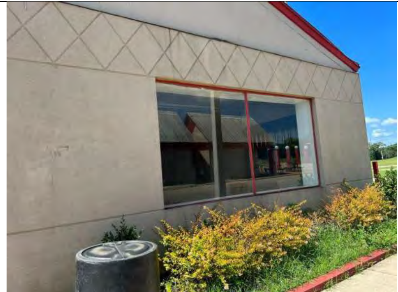
BUILDING 7 PHOTO #8: View of typical fixed window at south elevation.
