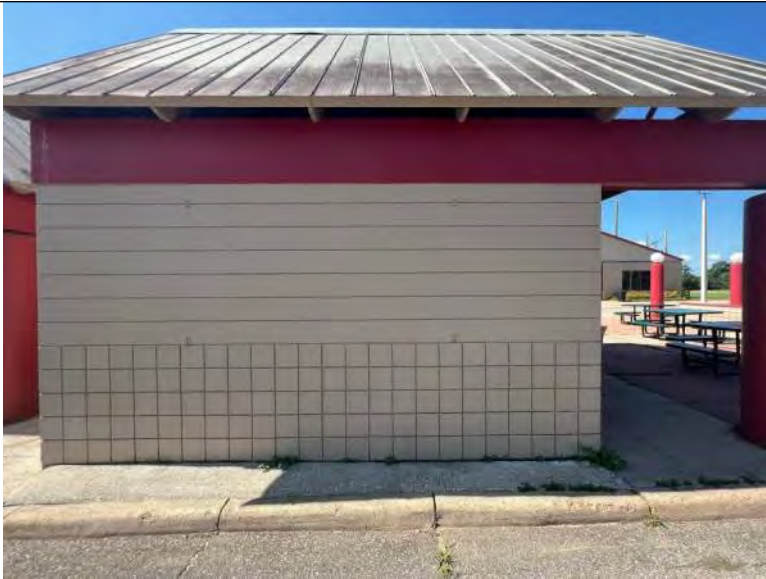
BUILDING C9-C11 PHOTO #5: Typical side elevation.
