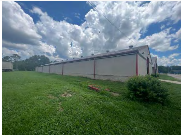
BUILDING 5 PHOTO #3: View of west elevation.
