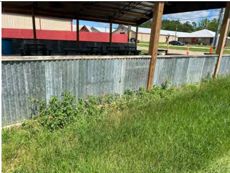
BUILDING 10 PHOTO #5: Corrugated metal paneling along bottom of structure side elevations.
