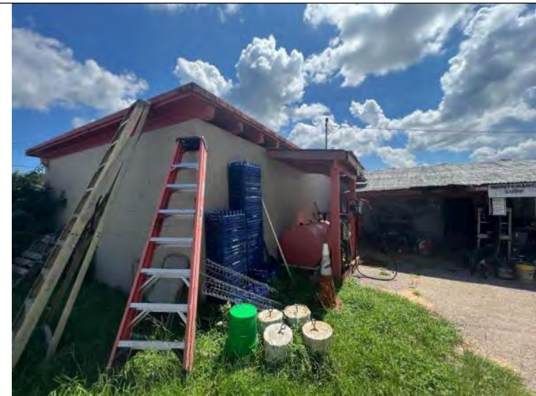
BUILDING R3 PHOTO #4: Partial view of west and south elevations.
