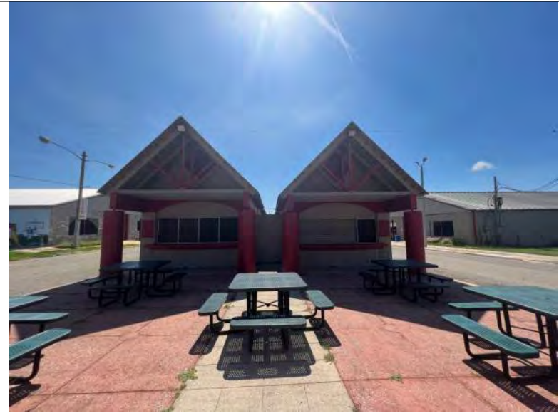
BUILDING C1-C4 PHOTO #2: Overview of Buildings C1 and C3.
