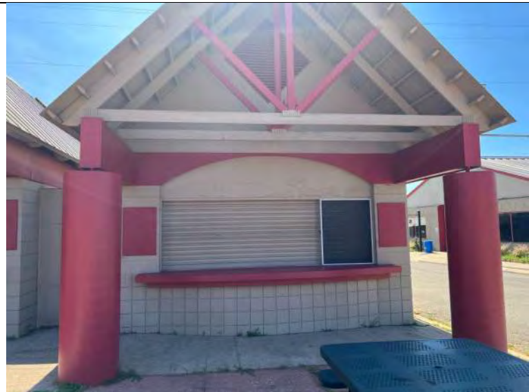
BUILDING C5-C8 PHOTO #3: Typical concrete masonry block construction, with concrete counter top and garage type door fenestration with screens of Buildings C1-C4.
