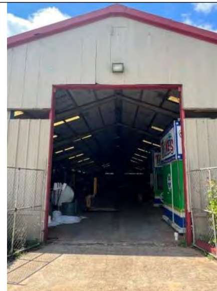
BUILDING 11 PHOTO #6: Overhead door opening on north elevation.
