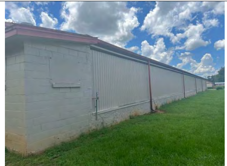
BUILDING 5 PHOTO #4: View of east elevation.
