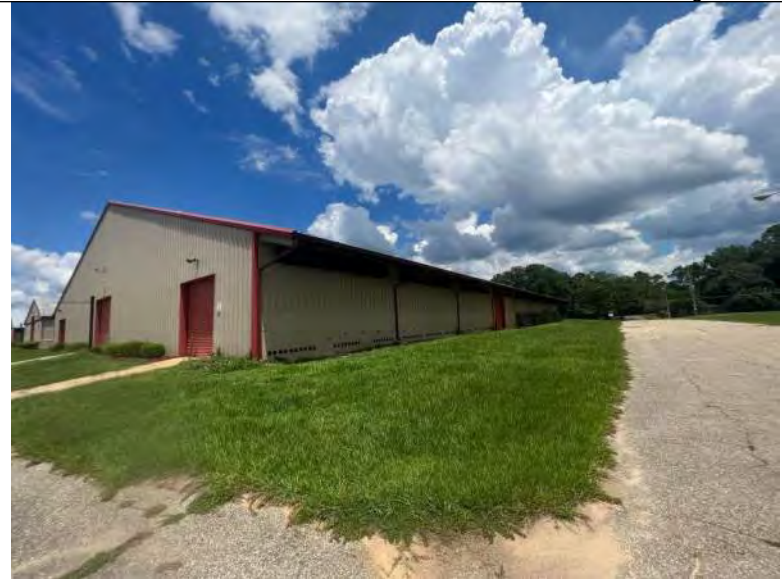
BUILDING 6 PHOTO #6: View of east elevation.
