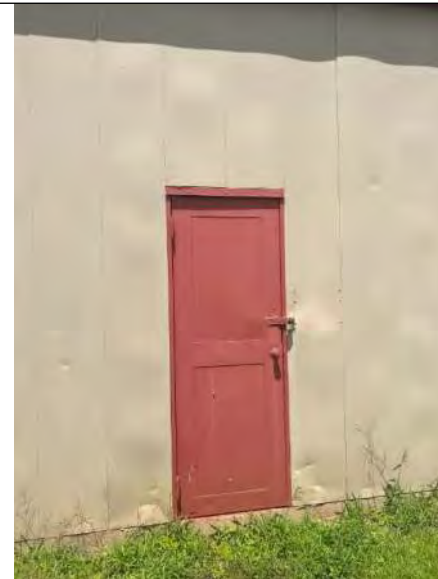
BUILDING 1 PHOTO #8: Typical service door.
