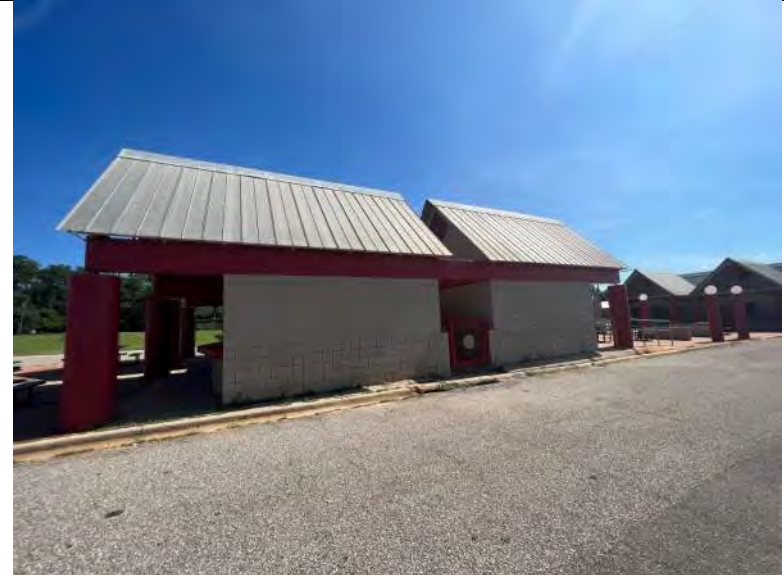
BUILDING C5-C8 PHOTO #6: Typical side elevations.
