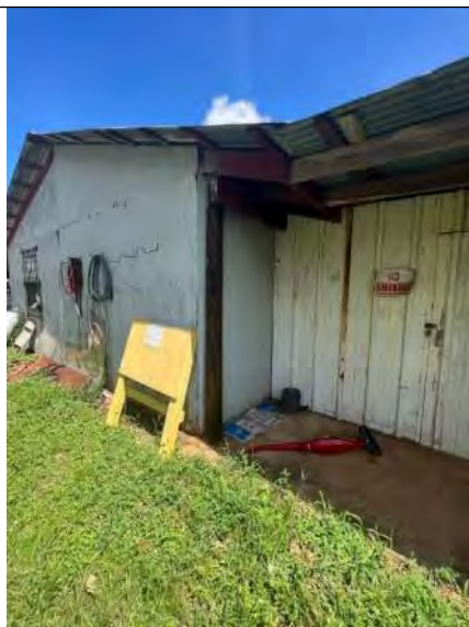
BUILDING M1 PHOTO #3: View of south elevation.
