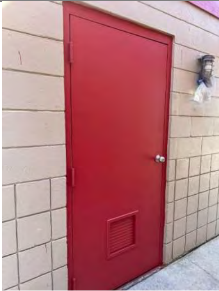
BUILDING C5-C8 PHOTO #9: Rear entry door to concessions buildings.
