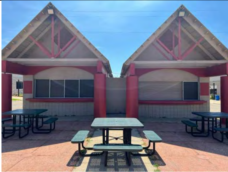
BUILDING C5-C8 PHOTO #1: Overview of Buildings C5-C7
