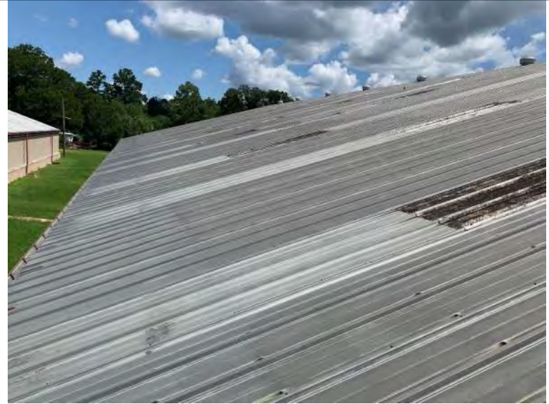
BUILDING 6 PHOTO #26: Overall view of metal roof panels associated with building 6.
