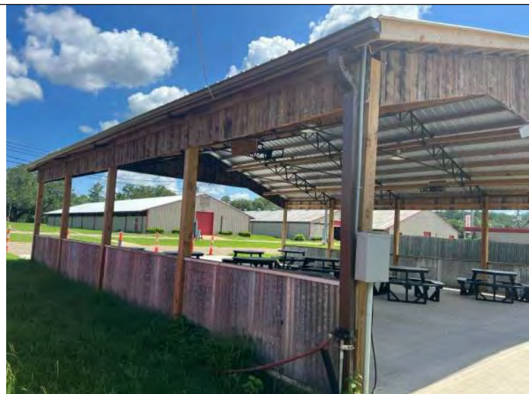
BUILDING 10 PHOTO #3: View of the west side of the structure.
