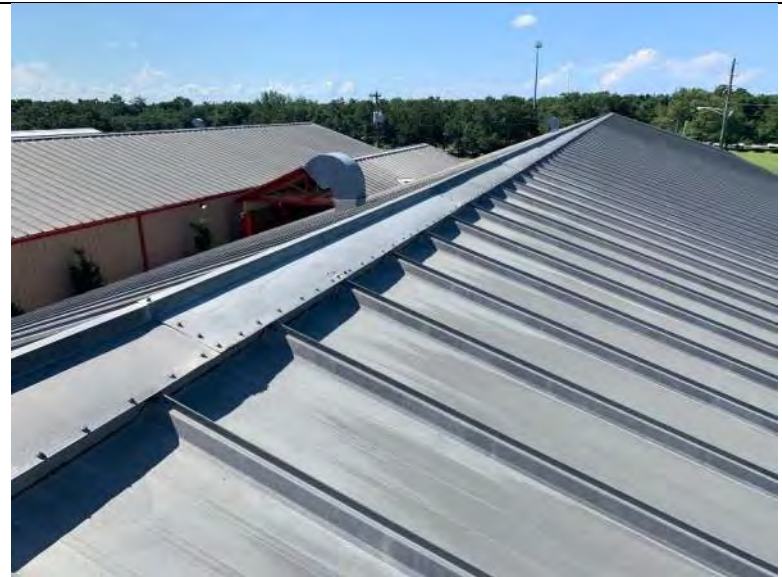
BUILDING 7 PHOTO #32: Vented metal ridge cap.
