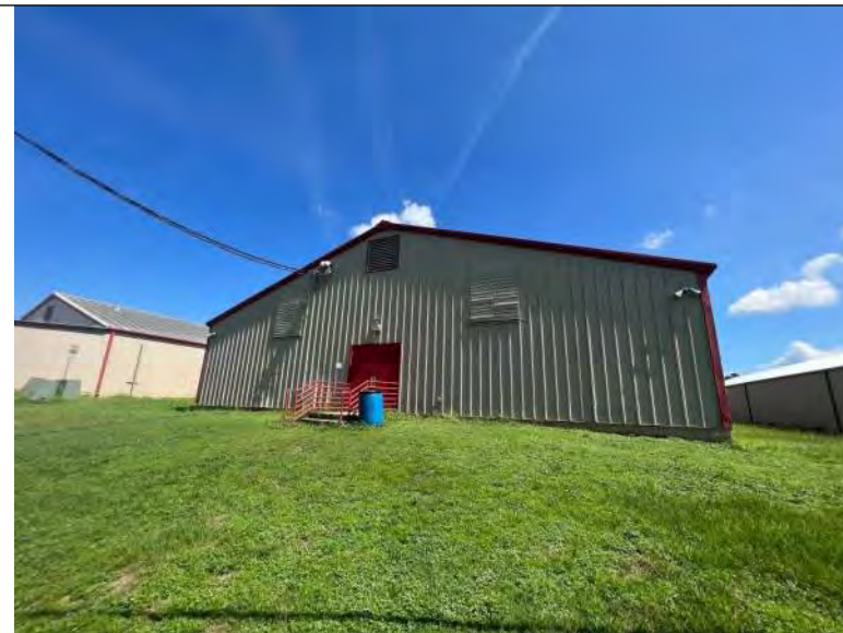
BUILDING 8 PHOTO #2: View of south elevation.
