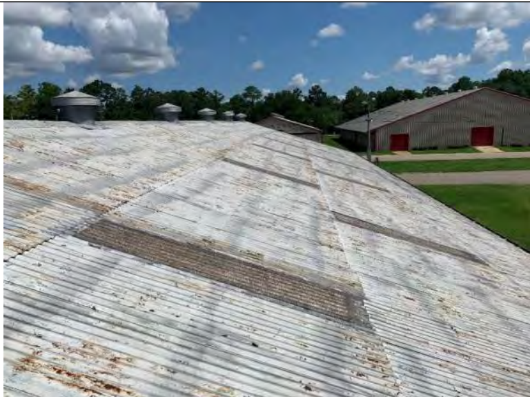
BUILDING 11 PHOTO #17: Translucent skylights located throughout roof area.
