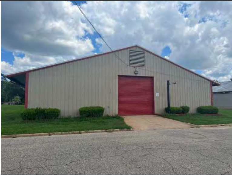
BUILDING 4 PHOTO #1: View of south elevation.
