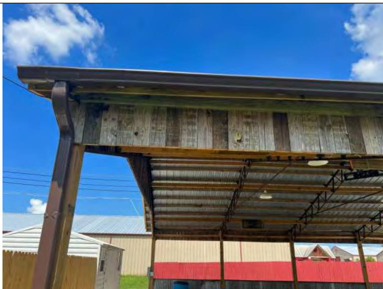
BUILDING 10 PHOTO #11: Wood planking at upper portions of structure.
