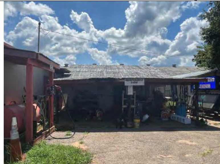
BUILDING M1 PHOTO #6: View of corrugated metal roofing.
