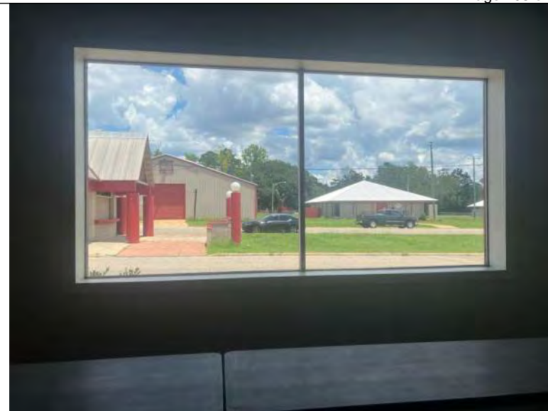
BUILDING 8 PHOTO #22: Interior view of fixed window.
