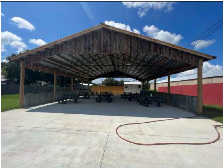
BUILDING 10 PHOTO #1: View of the north side of the structure.
