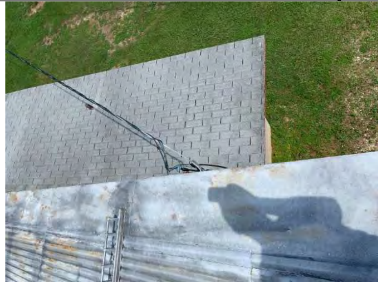
BUILDING 5 PHOTO #30: Shed with shingle roof system.
