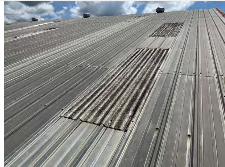
BUILDING 6 PHOTO #32: Translucent skylights located throughout roof area.
