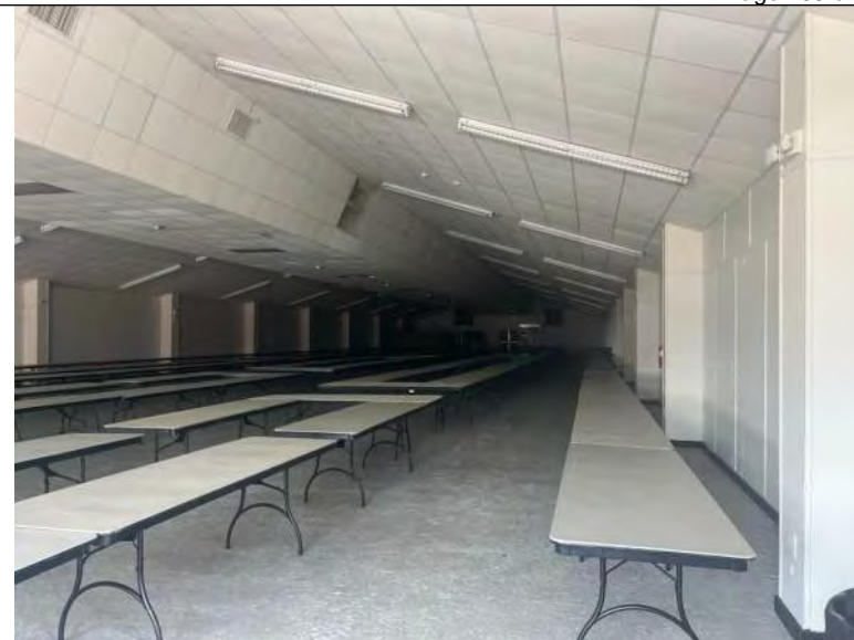
BUILDING 8 PHOTO #26: Interior view of Building 8.
