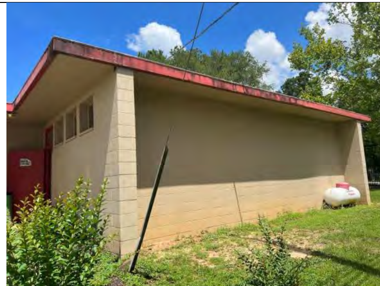
BUILDING R1 PHOTO #2: View of east elevation.
