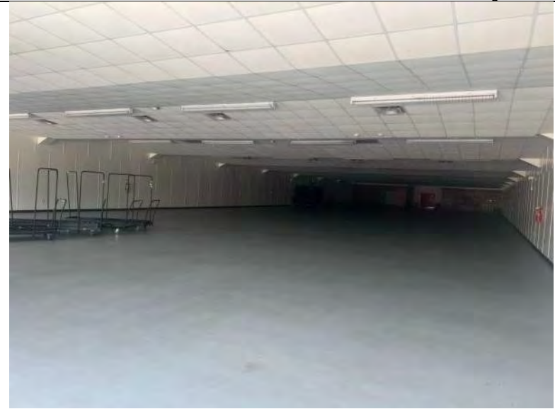
BUILDING 7 PHOTO #10: View of interior.
