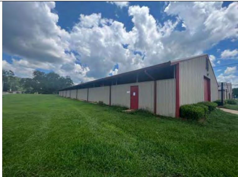
BUILDING 4 PHOTO #3: View of west elevation.
