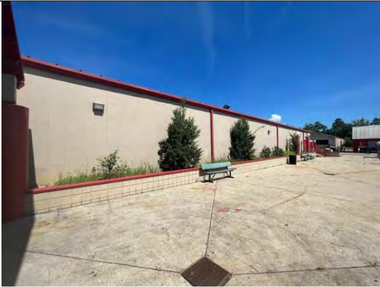
BUILDING 7 PHOTO #5: Partial view of east elevation
