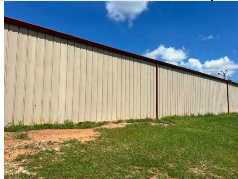
BUILDING 9 PHOTO #6: Partial view of east elevation
