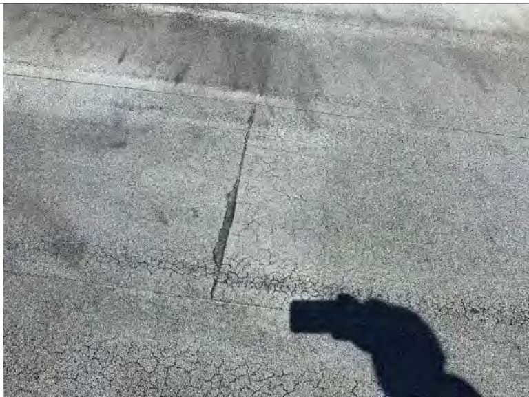
BUILDING R3 PHOTO #9: Overall view of modified bitumen BUR with granular cap sheet associated with building R3.
