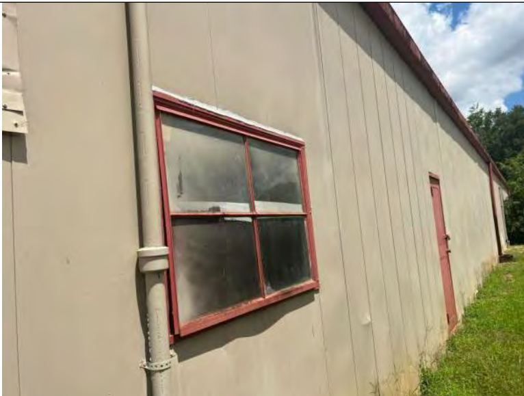
BUILDING 1 PHOTO #7: Typical operable window system.
