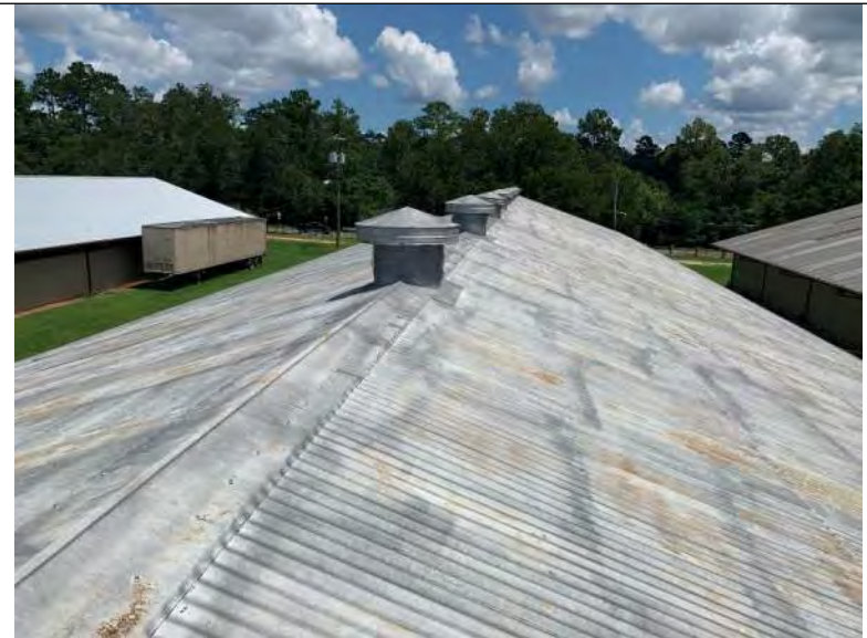
BUILDING 5 PHOTO #24: Metal ridge cap.
