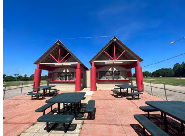
BUILDING C5-C8 PHOTO #2: Overview of Buildings C6 and C8.
