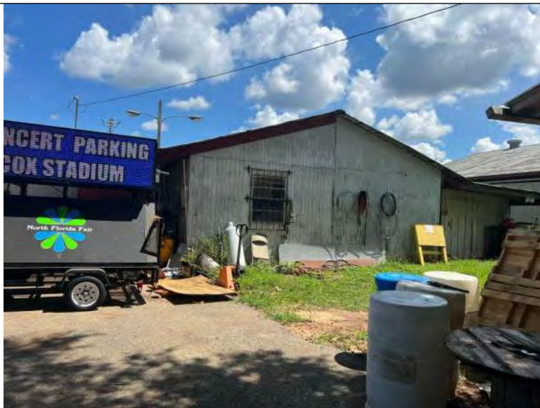
BUILDING M1 PHOTO #1: View of maintenance structure south elevation
