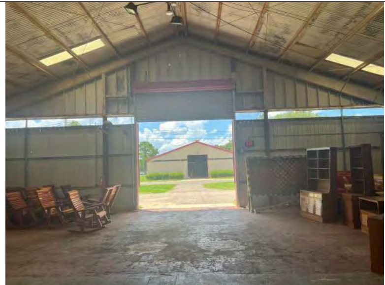
BUILDING 6 PHOTO #12: Interior view of Building 6.
