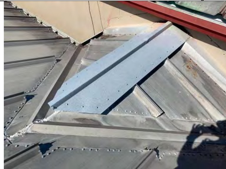
BUILDING R2 PHOTO #10: Transition between building R2 and building 7.
