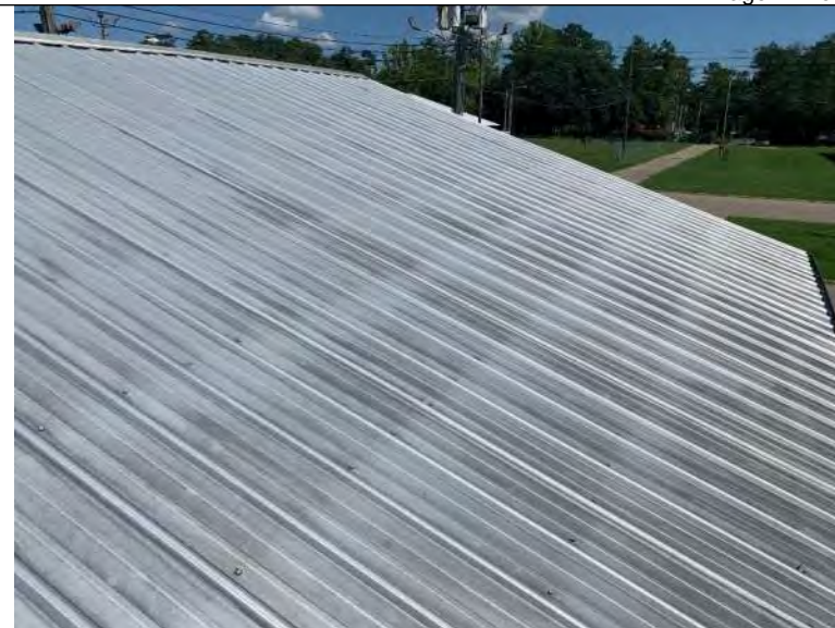
BUILDING 10 PHOTO #14: Overall view of metal roof panels associated with building 10.
