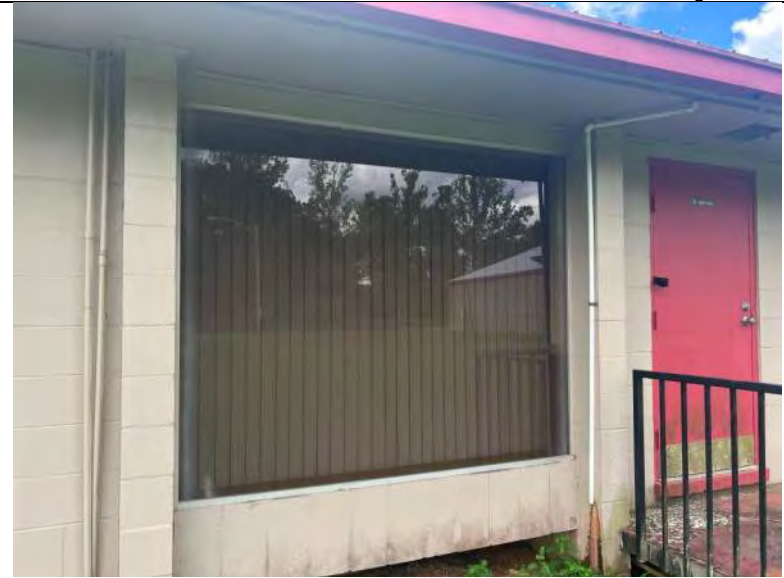
BUILDING 3 PHOTO #6: Typical picture window observed.
