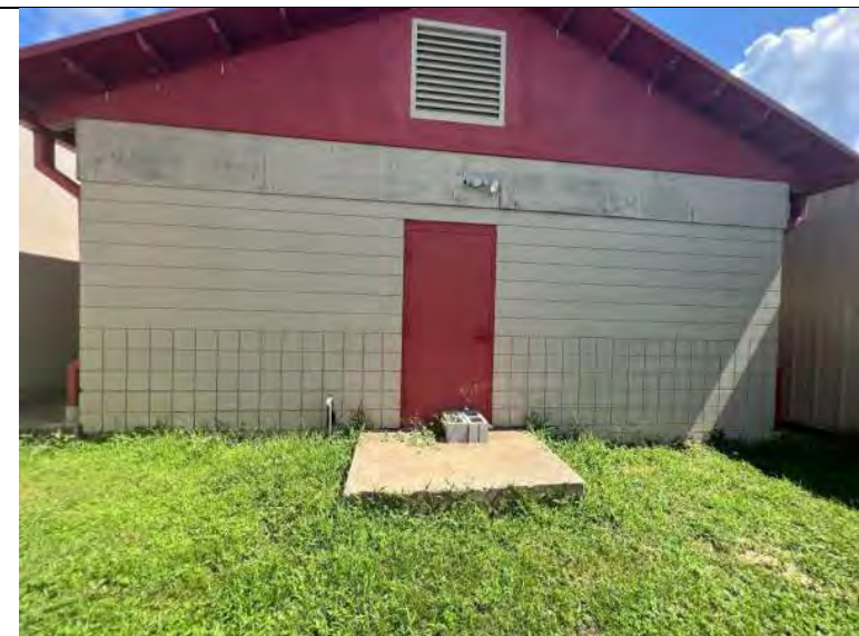
BUILDING R2 PHOTO #4: View of south elevation.
