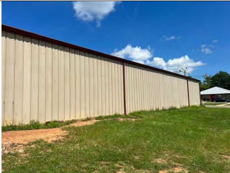
BUILDING 9 PHOTO #5: Partial view of east elevation.
