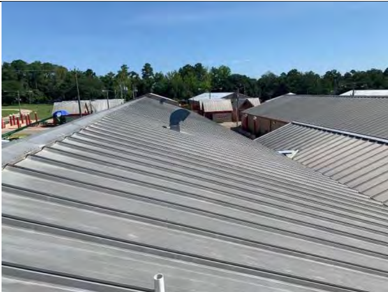
BUILDING 7 PHOTO #31: Overall view of metal roof panels associated with building 7.
