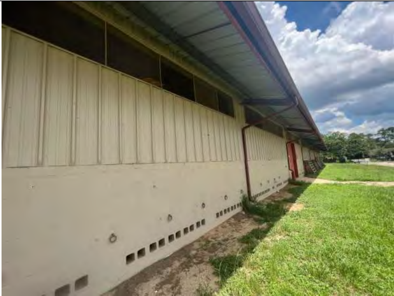
BUILDING 6 PHOTO #5: Partial view of east elevation.
