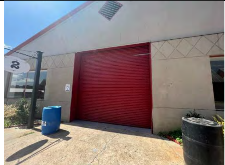
BUILDING 7 PHOTO #6: View of overhead door at south elevation.
