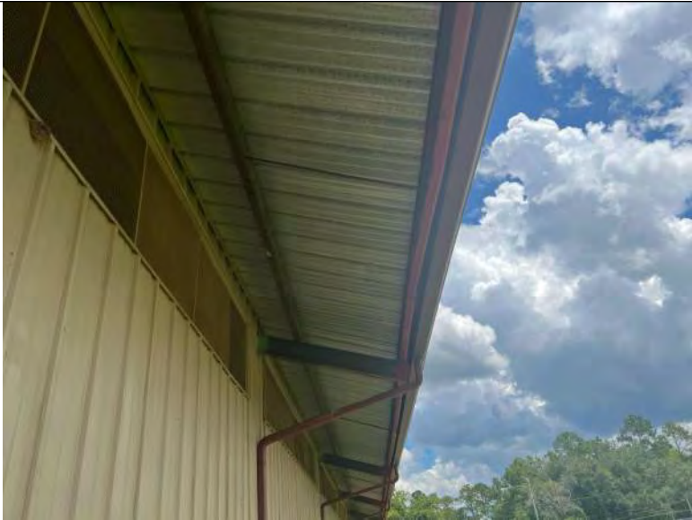
BUILDING 6 PHOTO #17: View of roof overhang.
