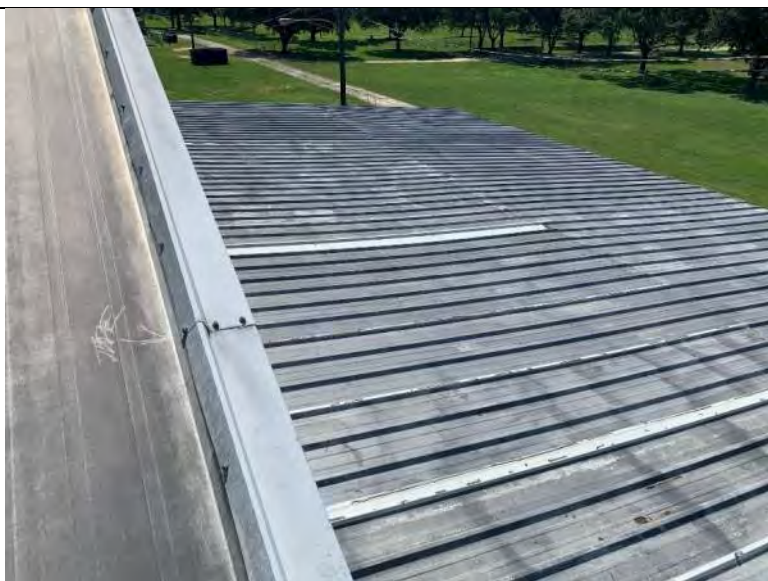
BUILDING 7 PHOTO #43: Metal roof covering shed on south elevation of building 7.
