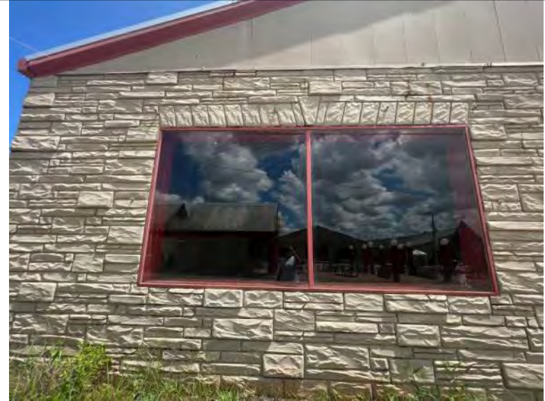
BUILDING 1 PHOTO #6: Typical inoperable window system.
