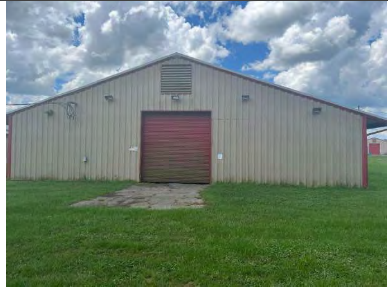
BUILDING 4 PHOTO #2: View of north elevation.
