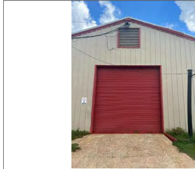
BUILDING 2 PHOTO #6: Overhead door at south elevation.
