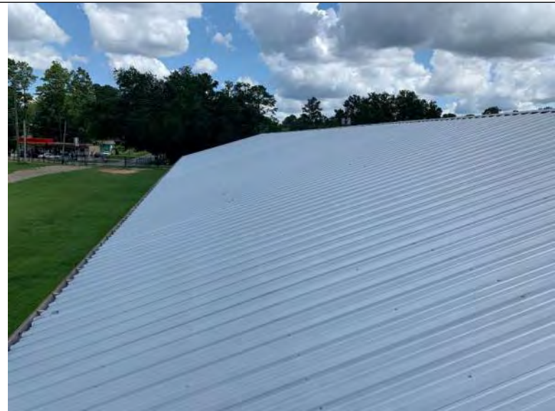
BUILDING 4 PHOTO #16: Overall view of metal roof panels associated with building 4.
