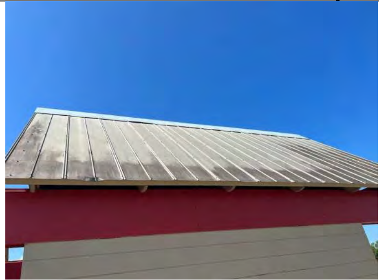
BUILDING C5-C8 PHOTO #10: Buildings C5-C8 have a metal panel roof system.
