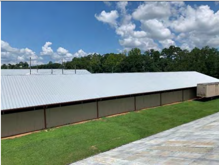
BUILDING 4 PHOTO #15: Overall view of metal roof panels associated with building 4.
