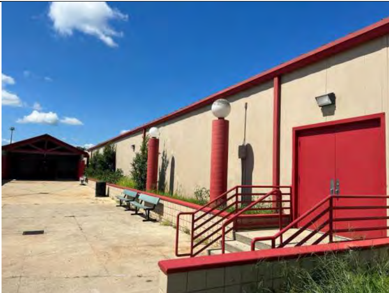
BUILDING 7 PHOTO #7: View of double service doors at east elevation.
