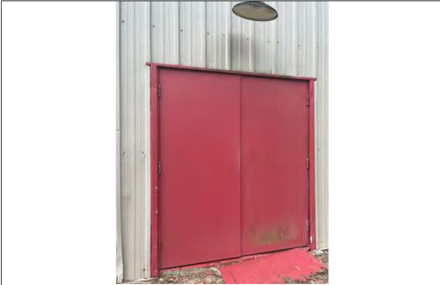
BUILDING 2 PHOTO #5: Service doors located at north elevation.
