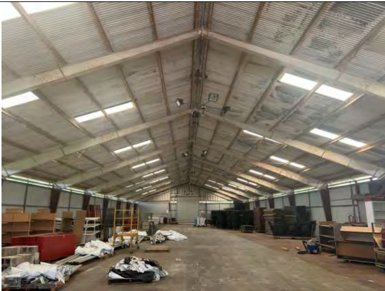
BUILDING 6 PHOTO #11: Interior view of Building 6.
