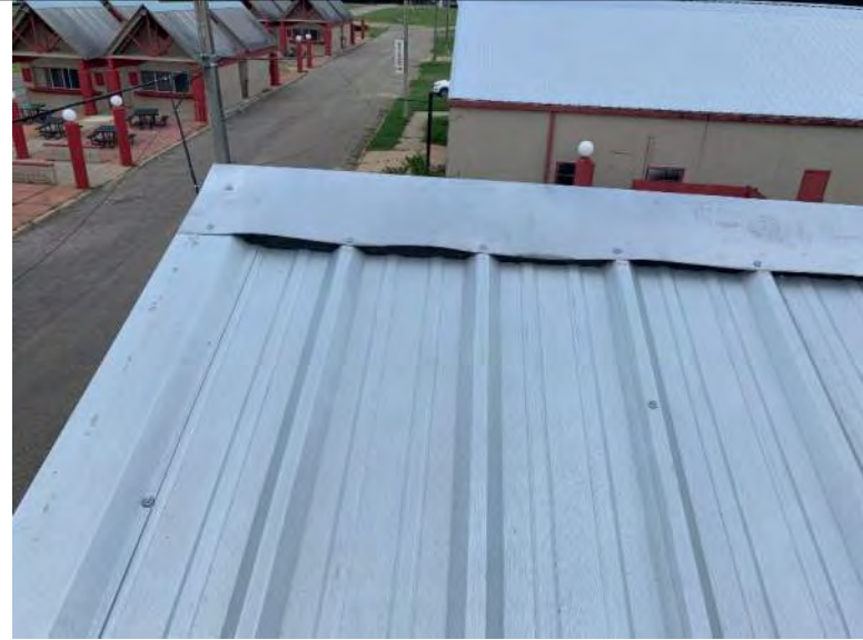
BUILDING 2 PHOTO #14: Metal ridge cap venting the building.
