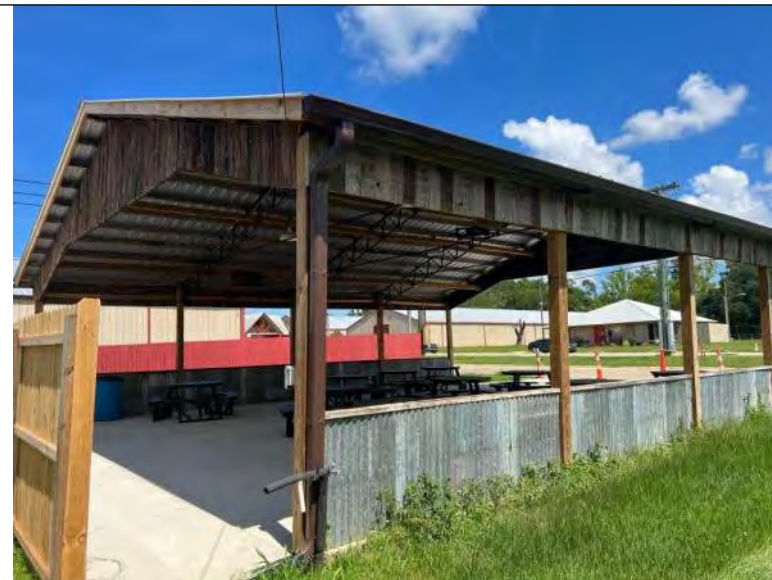
BUILDING 10 PHOTO #2: View of the east side of the structure.
