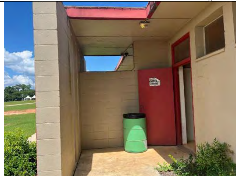
BUILDING R1 PHOTO #6: Typical metal door to restroom facilities.
