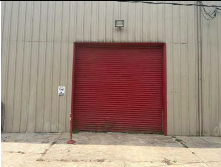
BUILDING 6 PHOTO #9: Overhead door at north elevation.
