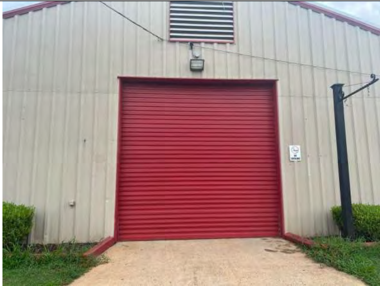
BUILDING 4 PHOTO #5: Overhead door on south elevation.
