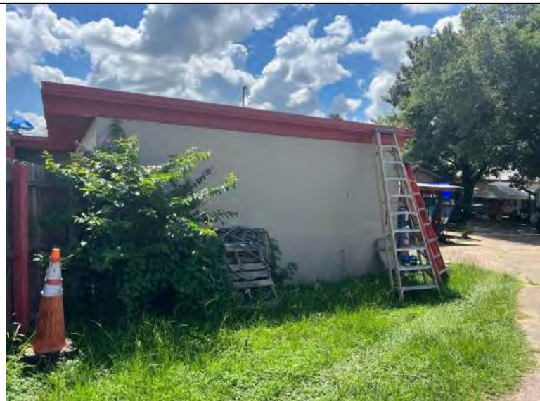
BUILDING R3 PHOTO #3: View of west elevation.
