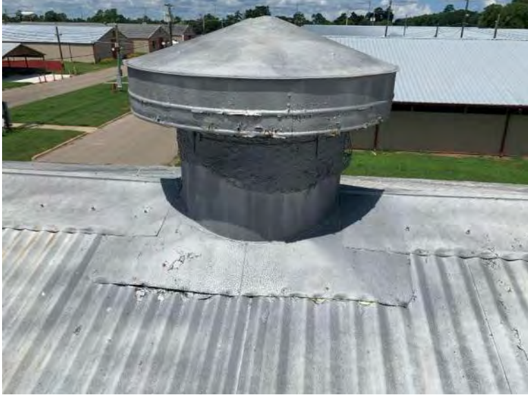
BUILDING 5 PHOTO #25: Roof penetrations include exhaust fans with metal flashing detail.
