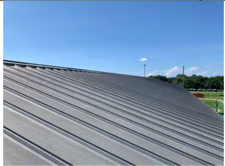
BUILDING 7 PHOTO #30: Overall view of metal roof panels associated with building 7.
