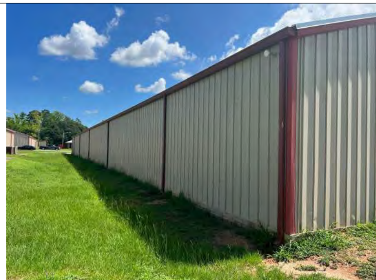
BUILDING 9 PHOTO #4: View of west elevation.
