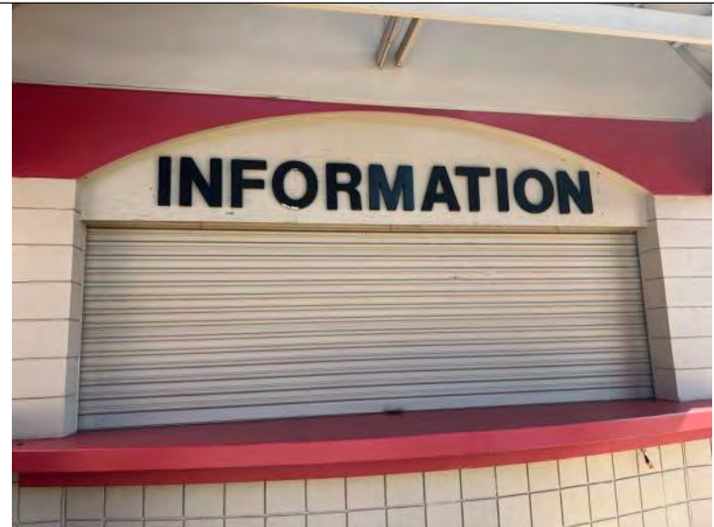
BUILDING C9-C11 PHOTO #12: Roll up door at information window.
