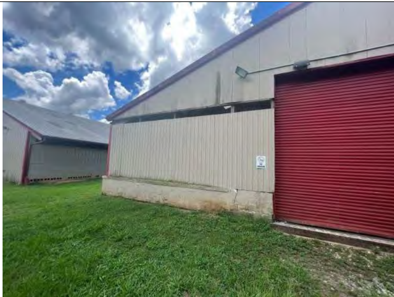
BUILDING 5 PHOTO #7: Overhead door at north elevation.
