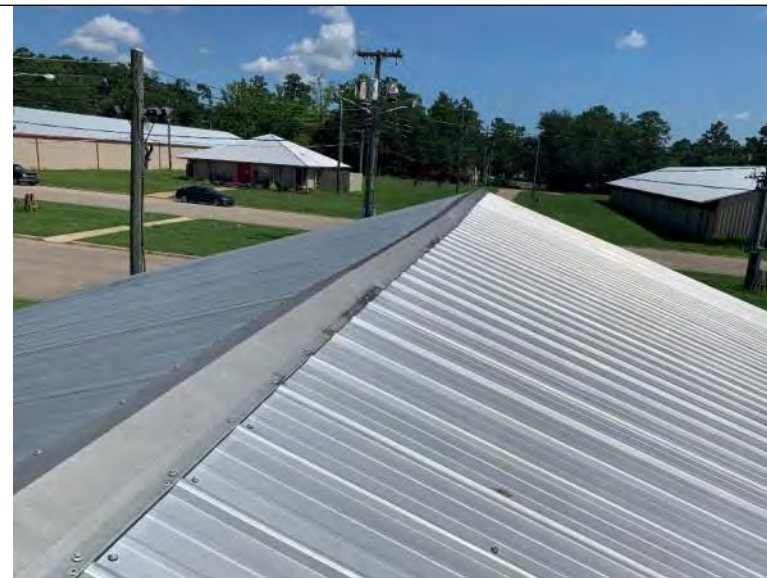
BUILDING 10 PHOTO #16: Metal ridge cap associated with building 10.
