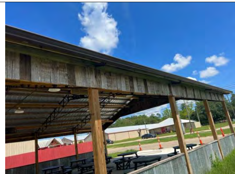
BUILDING 10 PHOTO #4: .View of the east side of the structure.
