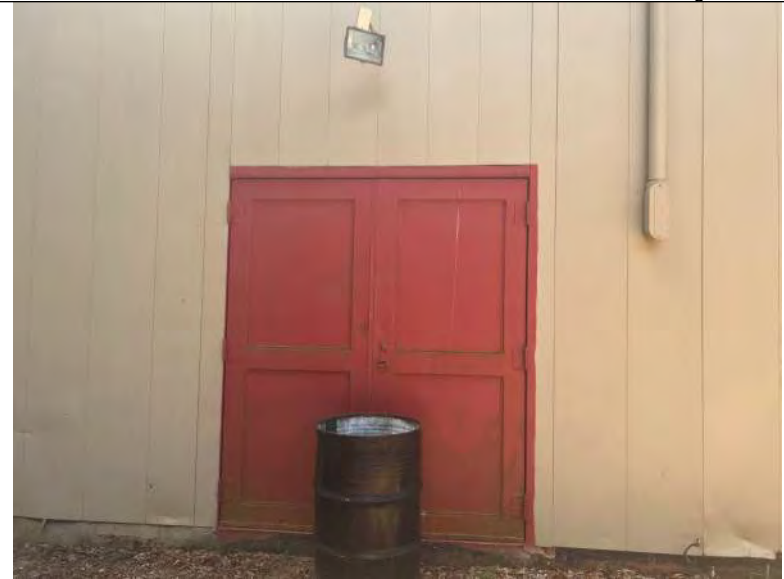
BUILDING 1 PHOTO #10: Double service door provided at north elevation.
