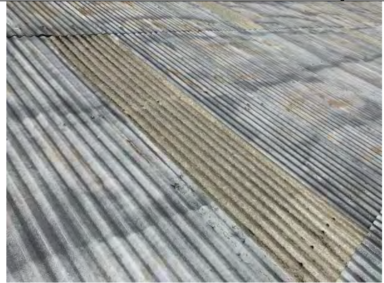
BUILDING 5 PHOTO #22: Translucent skylights located throughout roof area.
