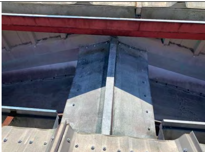
BUILDING R2 PHOTO #11: Transition between building R2 and building 8.
