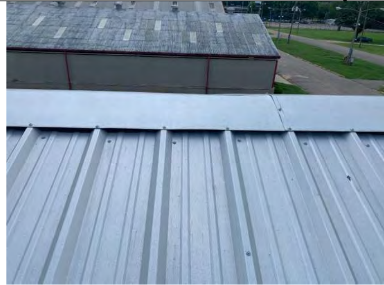
BUILDING 4 PHOTO #18: Vented metal ridge cap.
