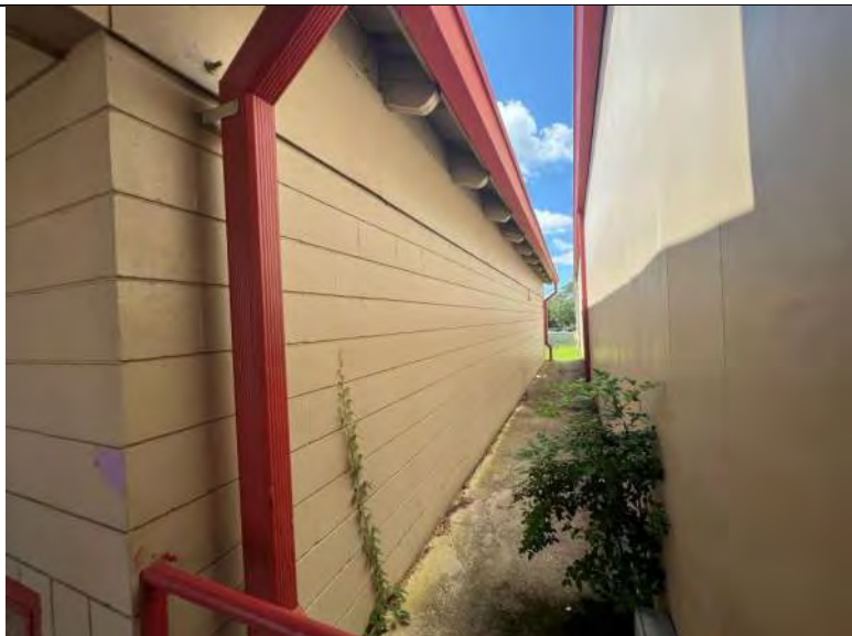
BUILDING R2 PHOTO #5: View of west elevation.
