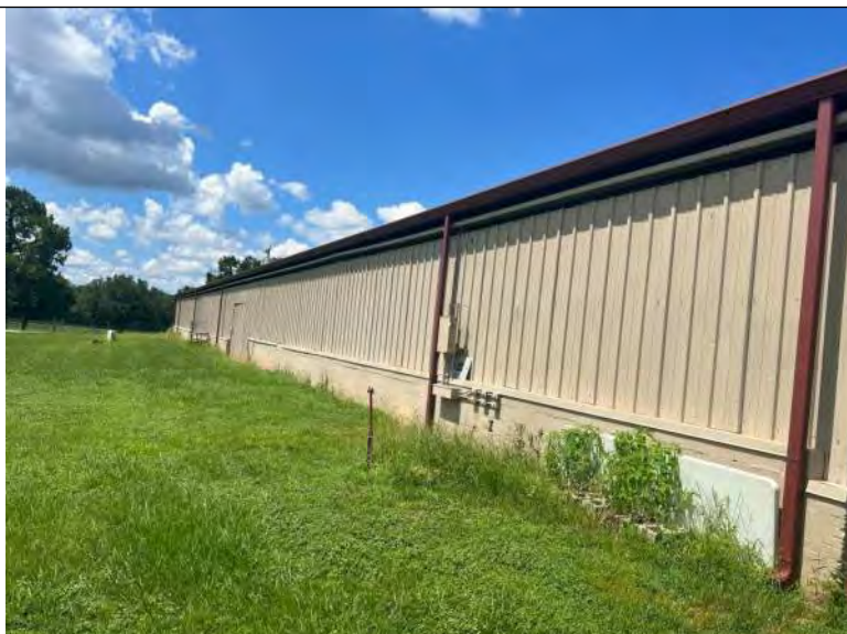
BUILDING 11 PHOTO #3: View of east elevation.
