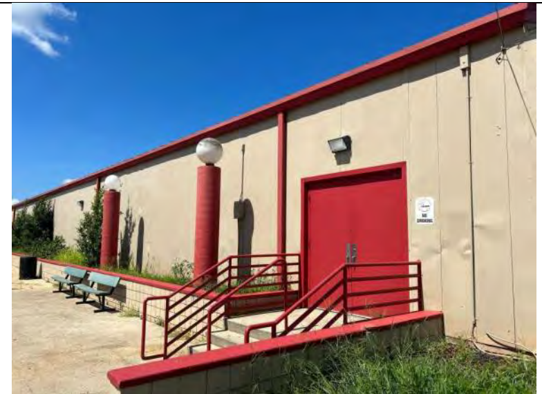
BUILDING 7 PHOTO #4: Partial view of east elevation.
