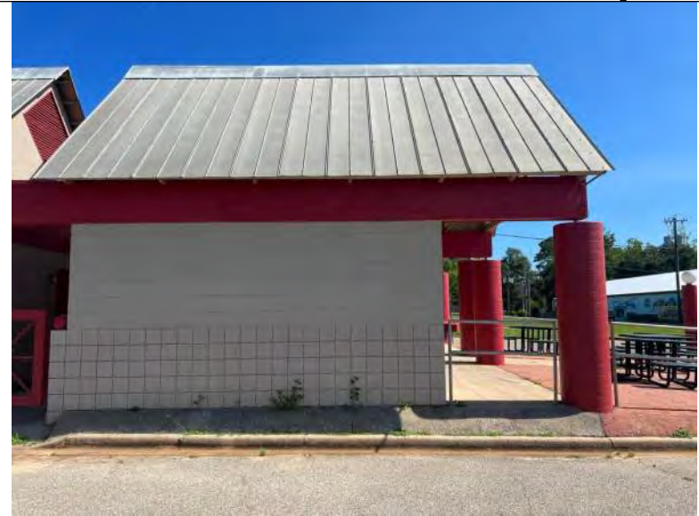
BUILDING C1-C4 PHOTO #6: Typical side elevation of Buildings C1-C4.
