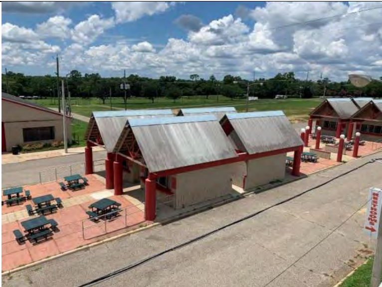
BUILDING C5-C8 PHOTO #15: Overall view of metal roof panels associated with buildings C5-C8.
