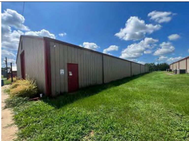
BUILDING 9 PHOTO #3: View of west elevation.
