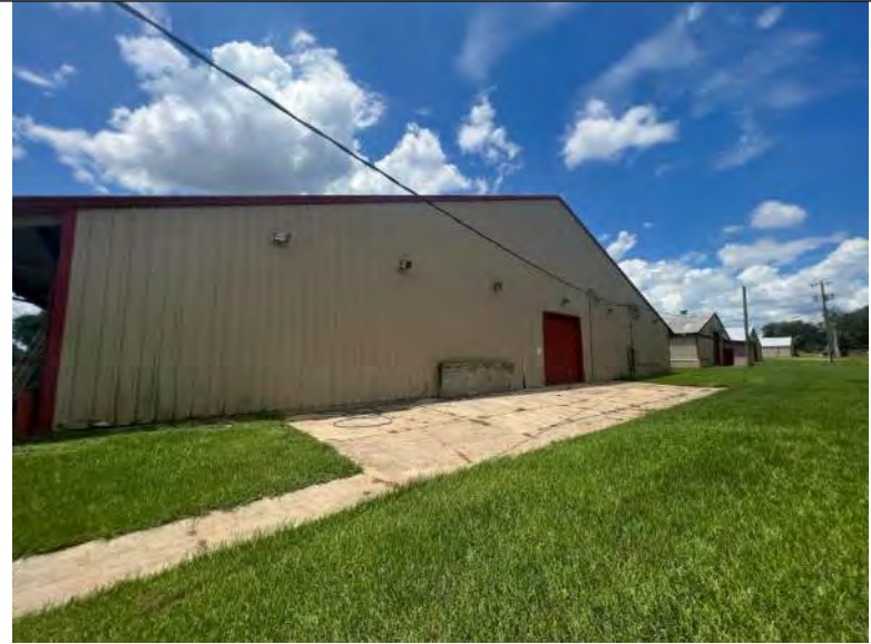
BUILDING 6 PHOTO #2: View of north elevation.
