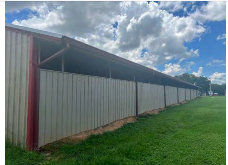
BUILDING 4 PHOTO #4: View of east elevation.
