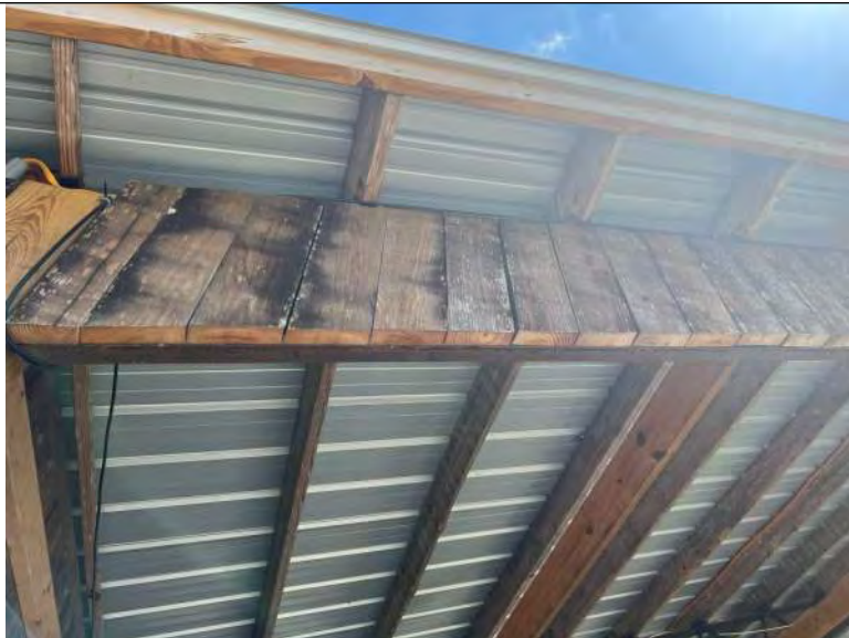
BUILDING 10 PHOTO #9: .Wood planking at upper portions of structure.
