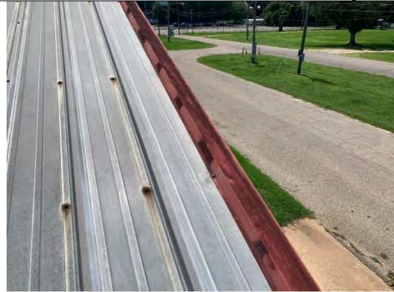
BUILDING 6 PHOTO #30: Roof perimeters consists of metal flashing.
