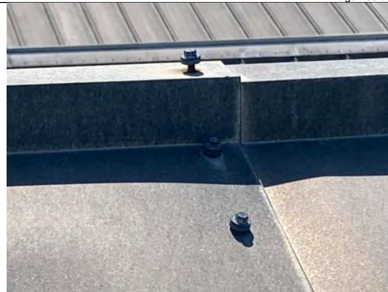
BUILDING 7 PHOTO #42: Withdrawing fasteners throughout roof area.
