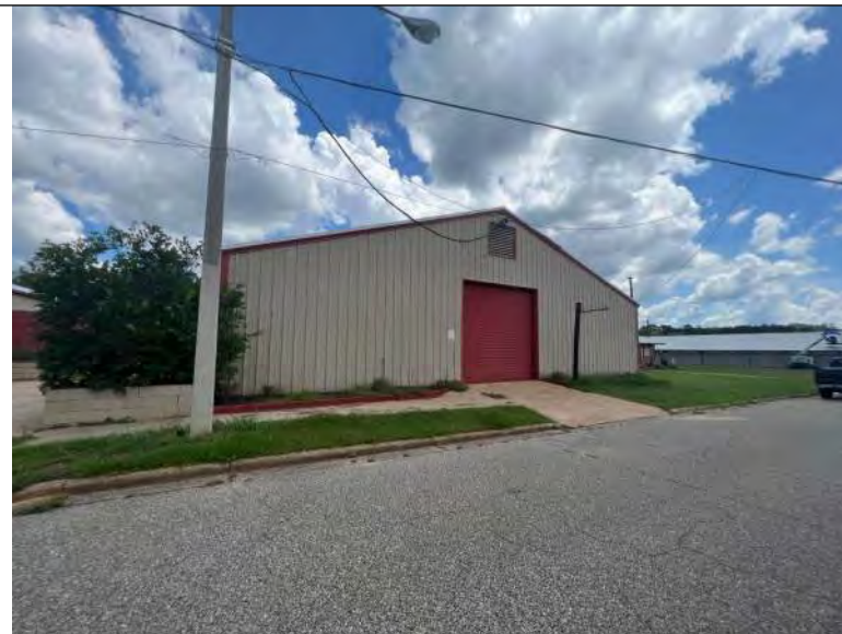
BUILDING 2 PHOTO #2: View of south elevation.
