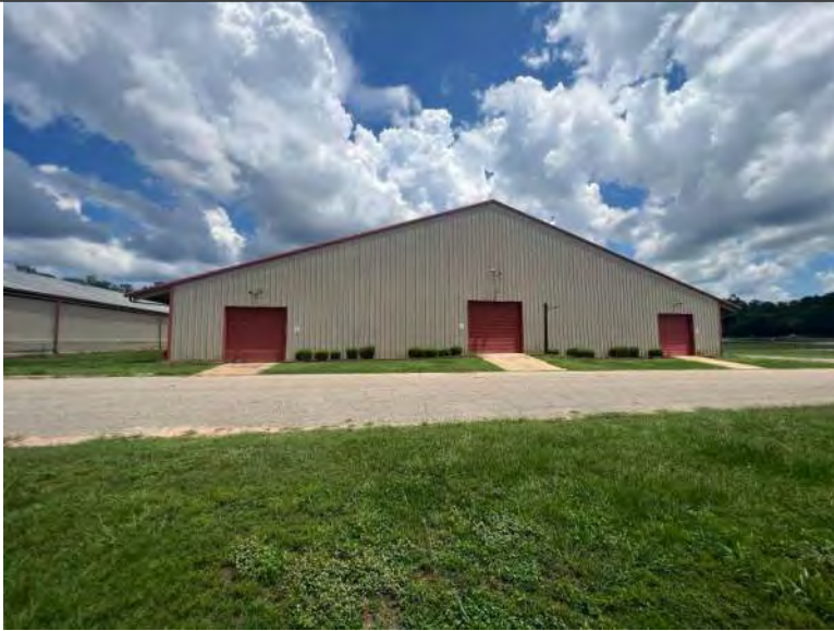
BUILDING 6 PHOTO #1: View of south elevation.
