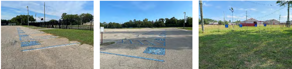
Figure 4.4.2 Existing Handicapped Parking ADA Assessment
