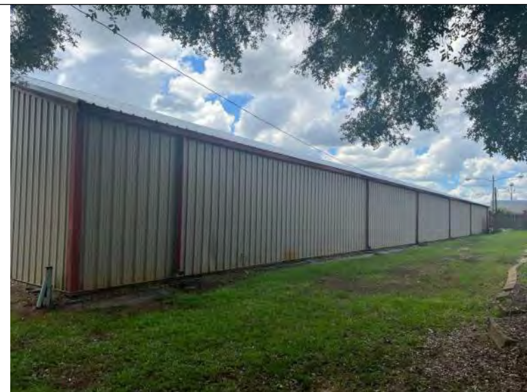
BUILDING 2 PHOTO #4: View of west elevation.
