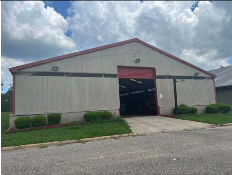
BUILDING 5 PHOTO #1: View of south elevation.
