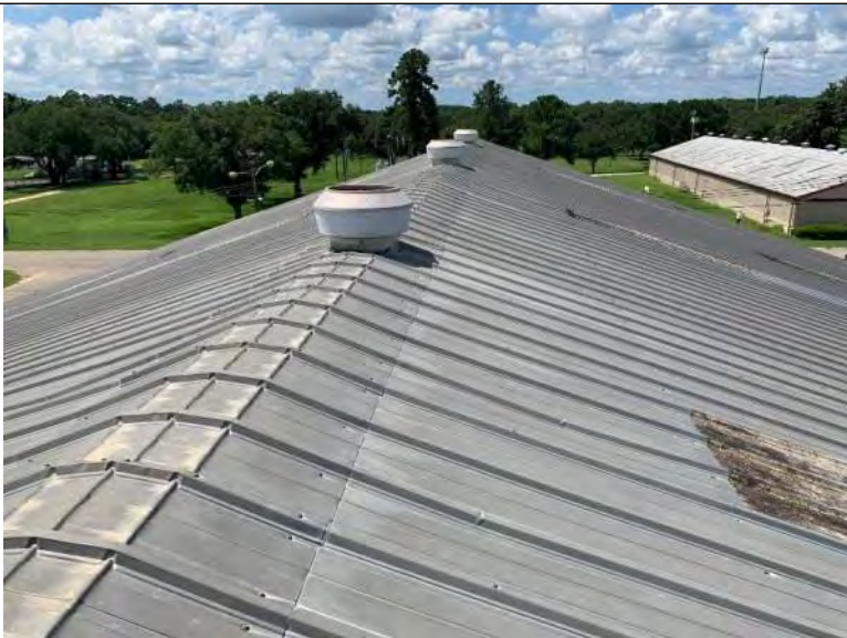
BUILDING 6 PHOTO #27: Metal ridge cap with exhaust fan roof penetrations.
