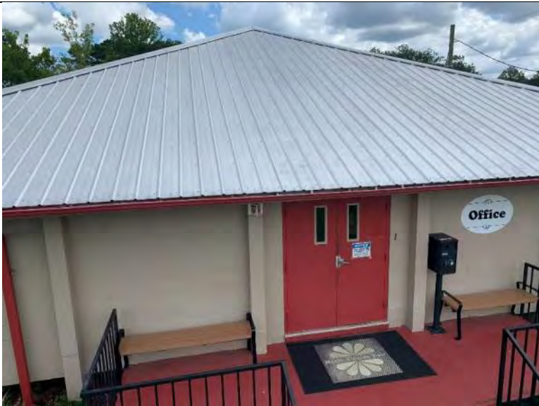
BUILDING 3 PHOTO #15: Overall view of metal roof panels associated with building 3.
