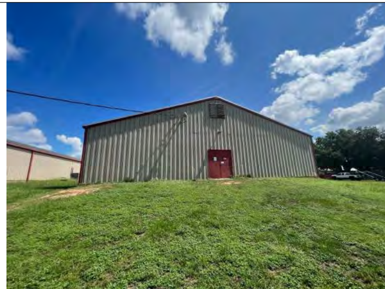
BUILDING 9 PHOTO #2: View of south elevation.
