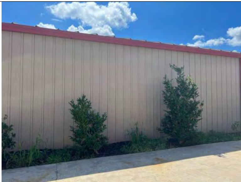
BUILDING 8 PHOTO #5: Partial view of west elevation.
