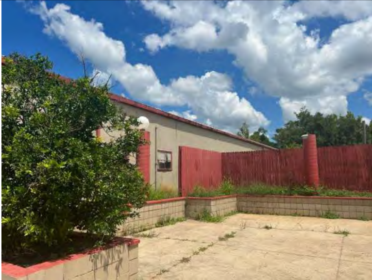
BUILDING 1 PHOTO #5: Partial view of east elevation.
