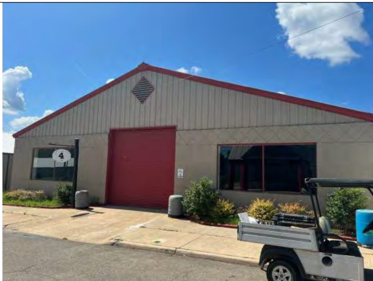
BUILDING 8 PHOTO #1: View of north elevation.
