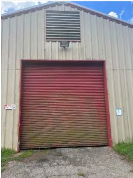
BUILDING 4 PHOTO #7: Overhead door on north elevation.
