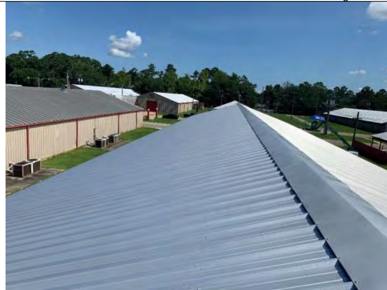
BUILDING 9 PHOTO #18: Overall view of metal roof panels associated with building 9.
