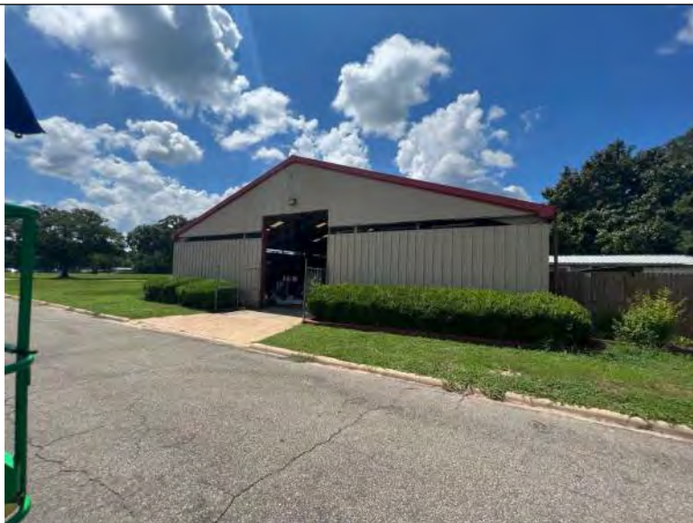
BUILDING 11 PHOTO #1: View of north elevation.
