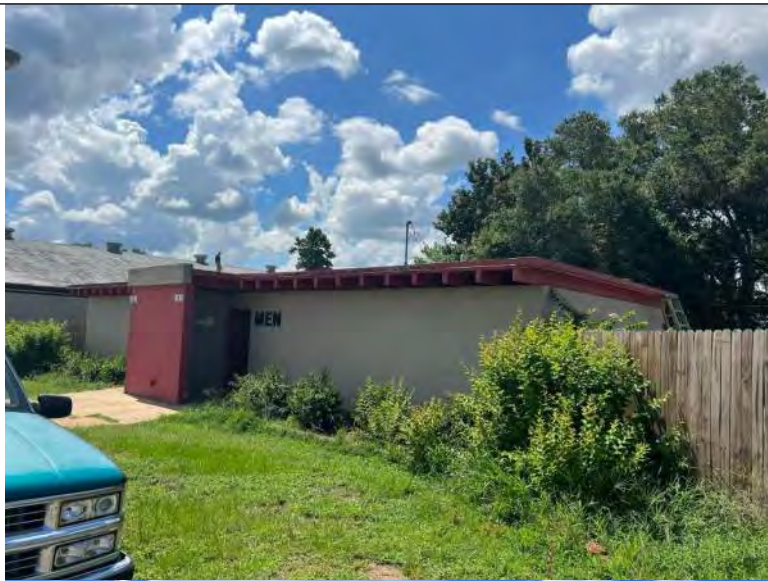
BUILDING R3 PHOTO #1: Partial View of north elevation.
