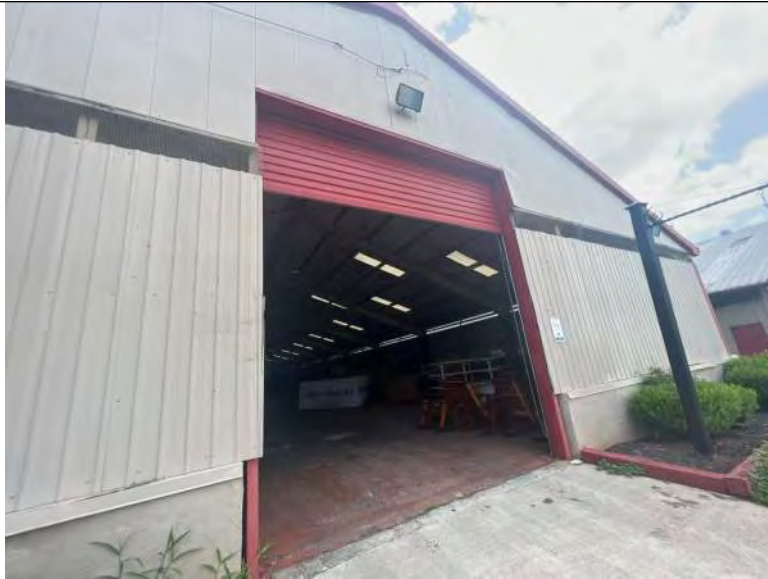
BUILDING 5 PHOTO #5: Overhead door at south elevation.
