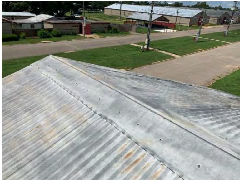
BUILDING 5 PHOTO #23: Metal ridge cap.
