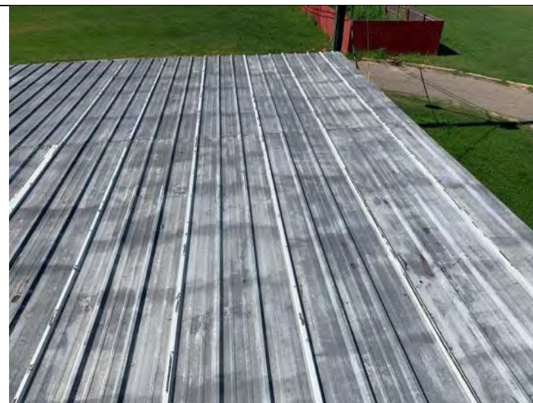
BUILDING 7 PHOTO #44: Metal roof covering shed on south elevation of building 7.
