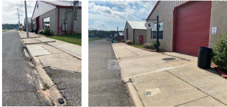
Figure 4.4.1 Existing Sidewalk ADA Assessment
