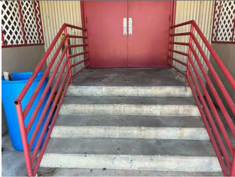
BUILDING 7 PHOTO #9: View of service door at north elevation.
