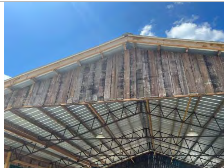
BUILDING 10 PHOTO #12: Wood planking at upper portions of structure.
