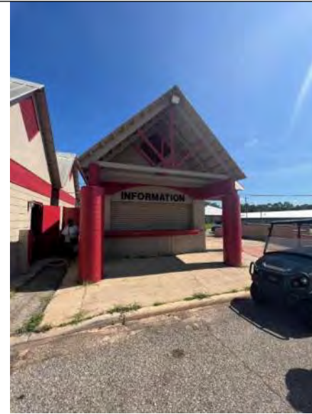
BUILDING C9-C11 PHOTO #2: Overview of Building C11.
