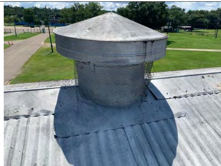
BUILDING 11 PHOTO #16: Exhaust fan roof penetrations flashed with metal detail.
