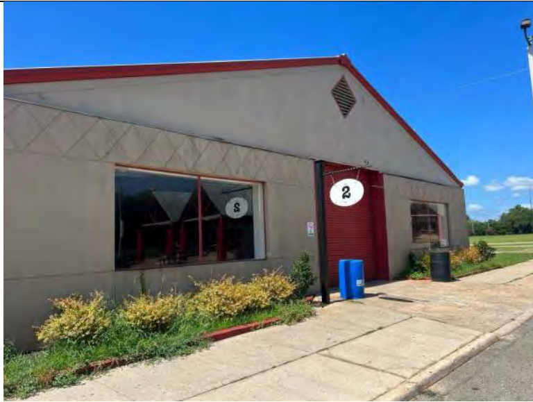
BUILDING 7 PHOTO #1: View of south elevation.
