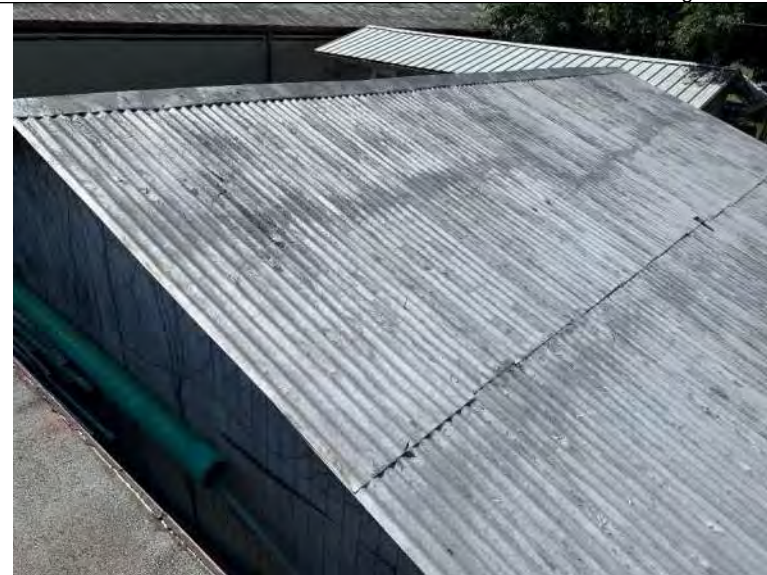
BUILDING M1 PHOTO #10: Metal ridge cap associated with building M3.
