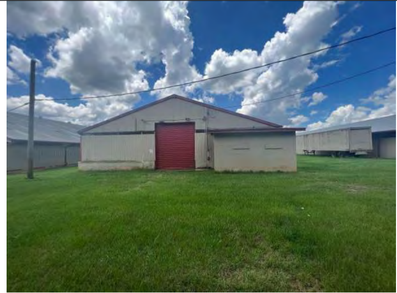
BUILDING 5 PHOTO #2: View of north elevation.
