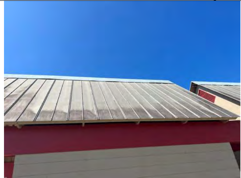
BUILDING C1-C4 PHOTO #10: Buildings C1-C4 have a metal panel roof system.
