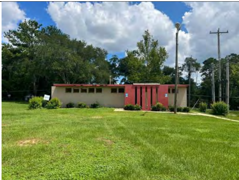
BUILDING R1 PHOTO #1: View of south elevation.
