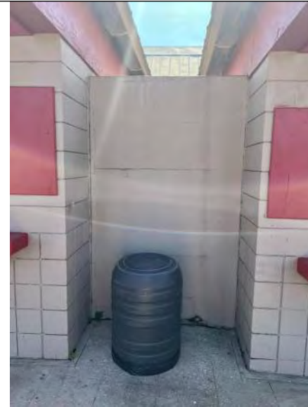
BUILDING C9-C11 PHOTO #6: CMU wall with stucco finish between buildings.
