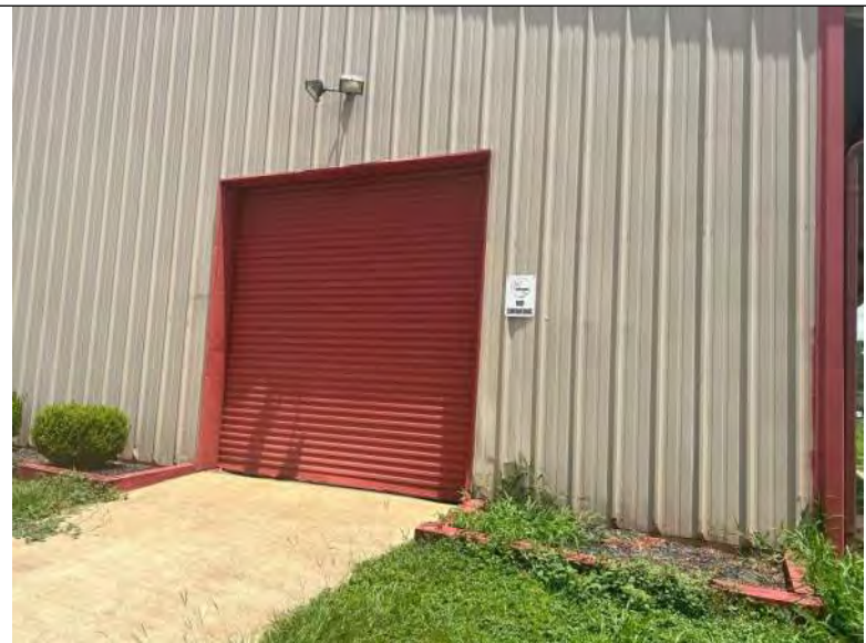
BUILDING 6 PHOTO #8: Overhead door at south elevation.
