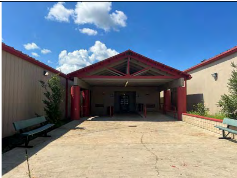
BUILDING R2 PHOTO #1: View of north elevation.
