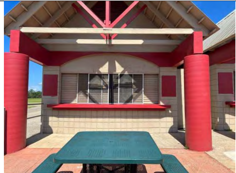
BUILDING C5-C8 PHOTO #8: Typical front elevation of Buildings C1-C4.
