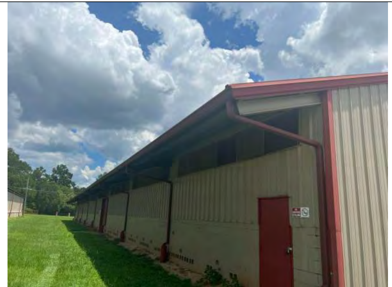
BUILDING 6 PHOTO #4: View of west elevation.
