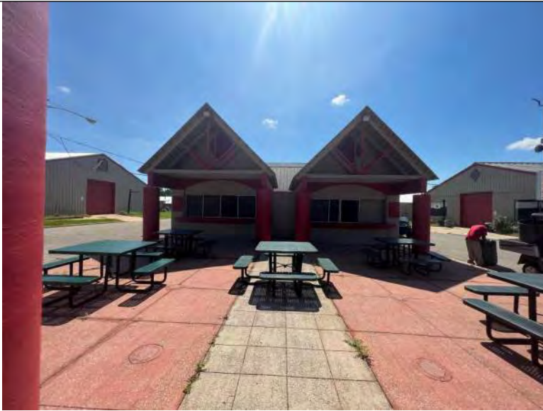
BUILDING C9-C11 PHOTO #1: Overview of Buildings C9 – C10.
