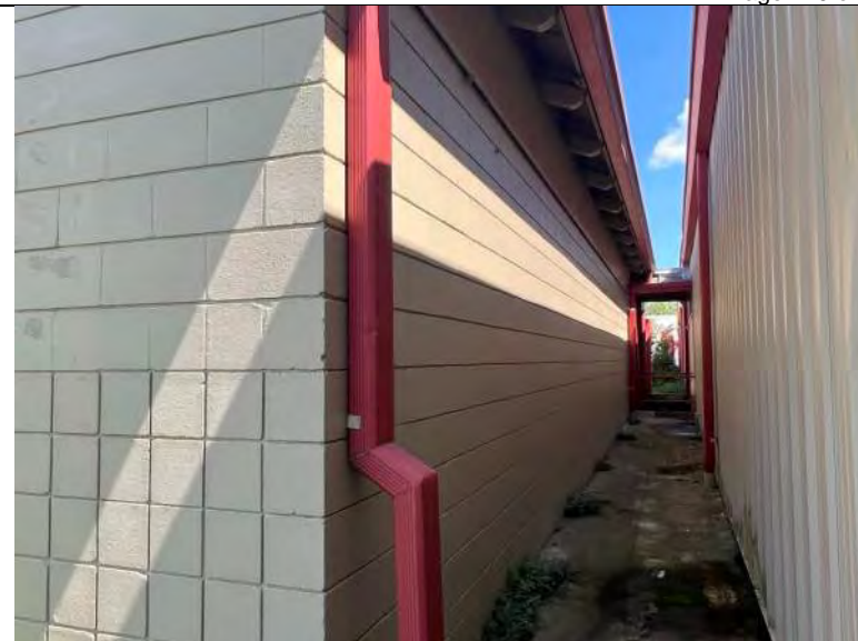
BUILDING R2 PHOTO #6: View of east elevation.
