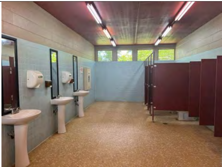
BUILDING R1 PHOTO #13: Interior view of men's restroom.
