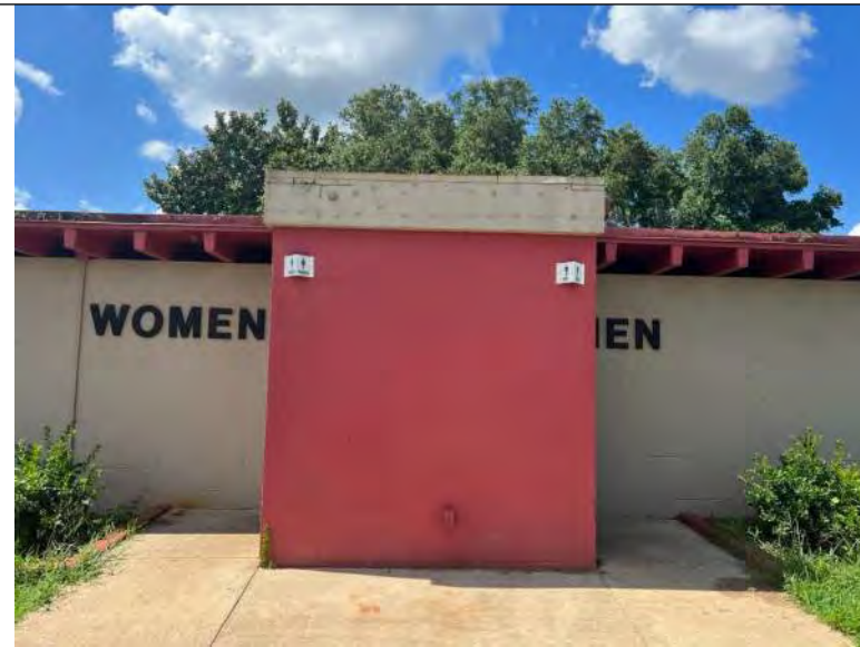
BUILDING R3 PHOTO #2: Partial View of north elevation.
