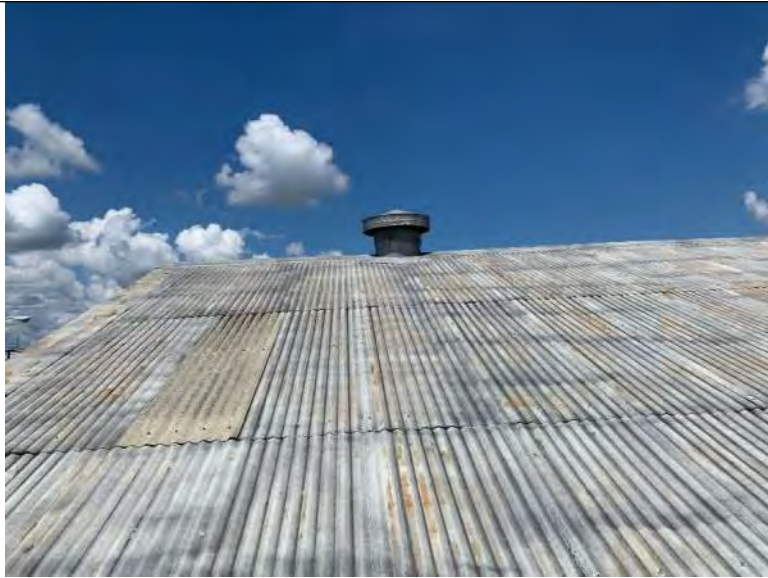
BUILDING 5 PHOTO #21: Translucent skylights located throughout roof area.
