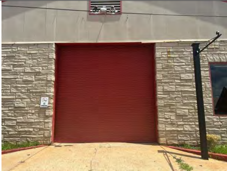
BUILDING 1 PHOTO #9: Overhead door provided on south elevation.
