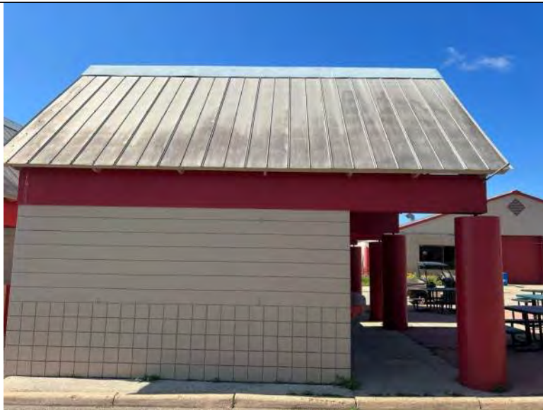
BUILDING C9-C11 PHOTO #11: The buildings have a metal panel roof system.
