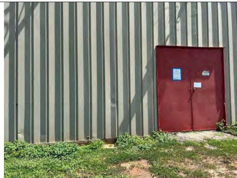
BUILDING 9 PHOTO #8: Typical double service door observed.
