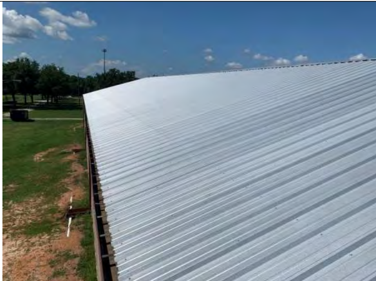
BUILDING 9 PHOTO #17: Overall view of metal roofing panels associated with building 9.
