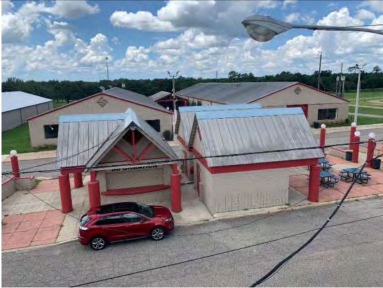
BUILDING C9-C11 PHOTO #13: Overall view of metal roof panels associated with buildings C9-C11.
