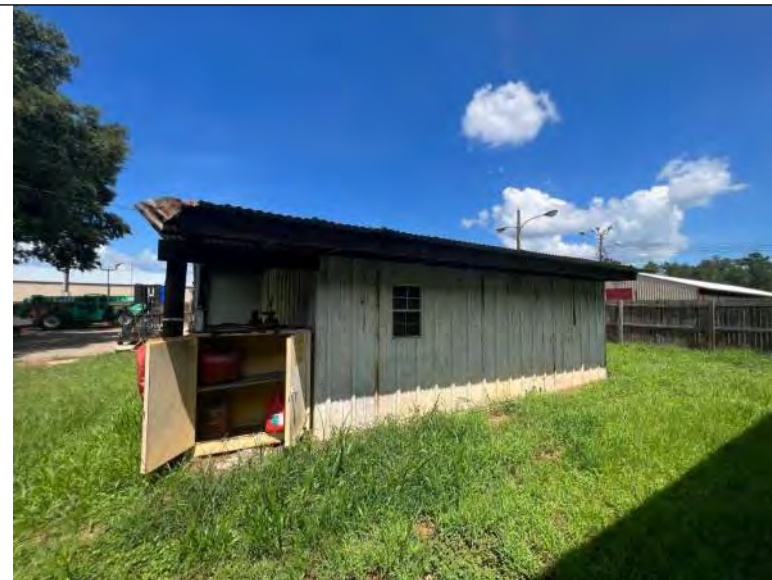
BUILDING M1 PHOTO #2: View of west elevation.
