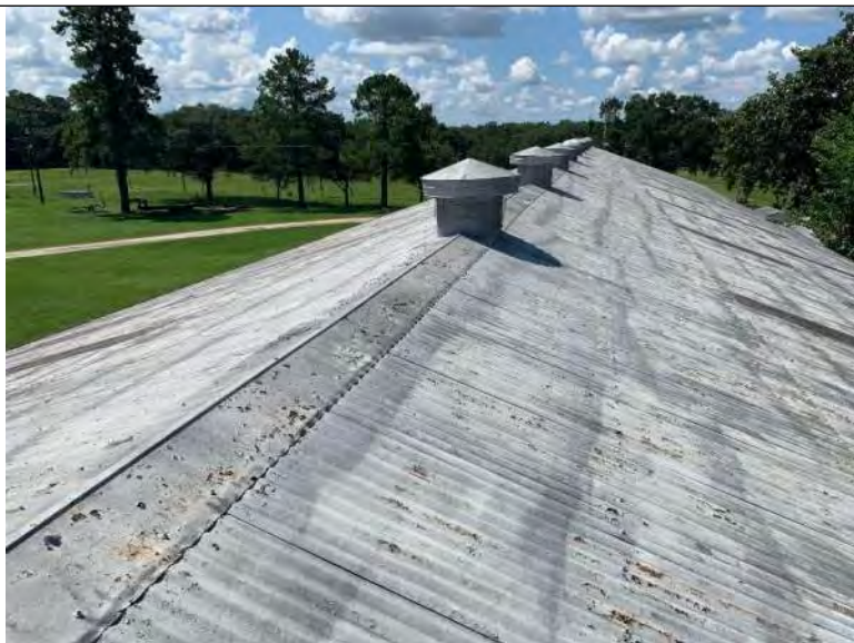
BUILDING 11 PHOTO #15: Metal ridge cap and exhaust fan roof penetrations.
