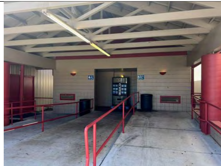
BUILDING R2 PHOTO #2: View of north elevation.
