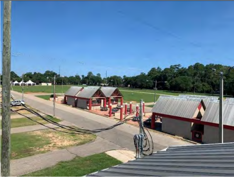
BUILDING C1-C4 PHOTO #21: Overall view of metal roof panels associated with buildings C1-C4.
