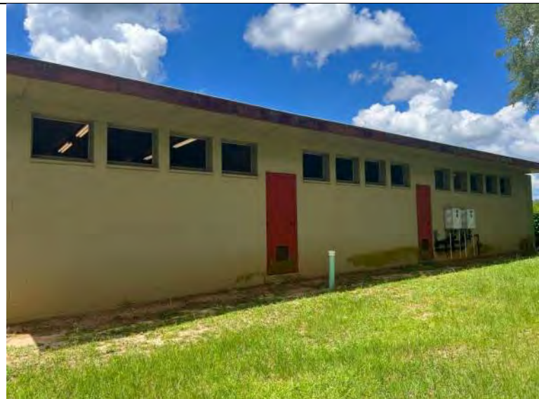
BUILDING R1 PHOTO #3: View of north elevation.
