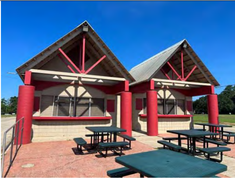
BUILDING C1-C4 PHOTO #1: Overview of Buildings C2 and C4.
