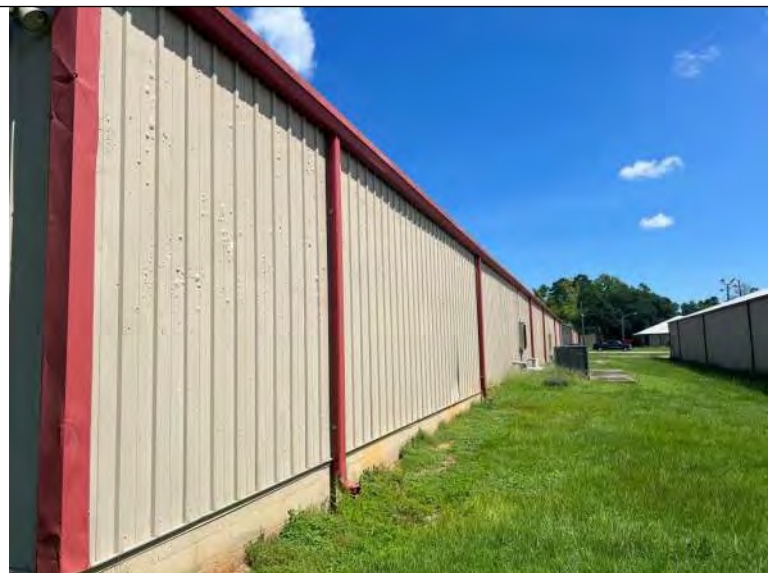
BUILDING 8 PHOTO #3: View of east elevation.
