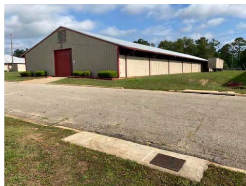
2) Drainage Inlets, Main Drive
