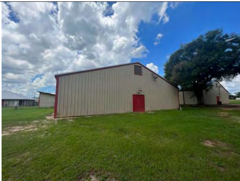
BUILDING 2 PHOTO #1: View of north elevation
