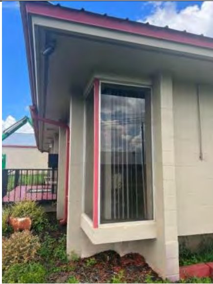
BUILDING 3 PHOTO #5: Typical corner window unit observed.
