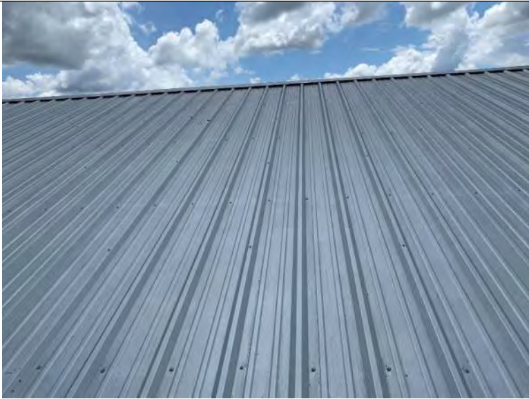
BUILDING 4 PHOTO #17: Exposed fasteners with neoprene washers.
