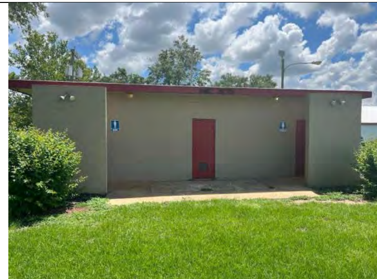
BUILDING R1 PHOTO #4: View of west elevation.
