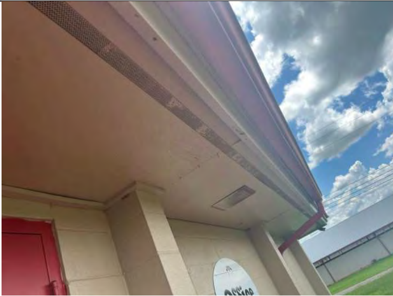
BUILDING 3 PHOTO #13: Typical soffit observed at building.
