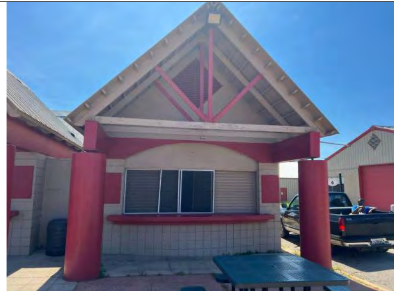
BUILDING C9-C11 PHOTO #8: Typical front elevation.
