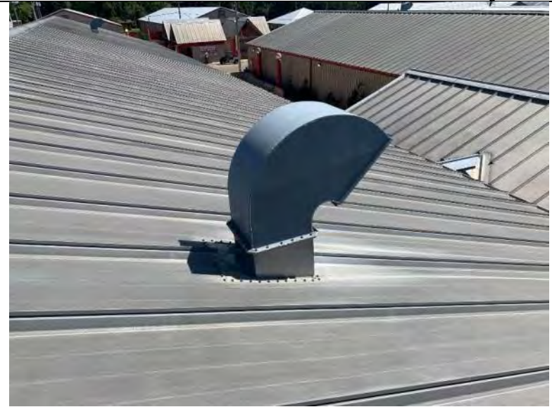
BUILDING 7 PHOTO #34: Roof penetrations include exhaust fans.
