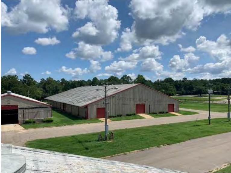
BUILDING 6 PHOTO #25: Overall view of metal roof panels associated with building 6.
