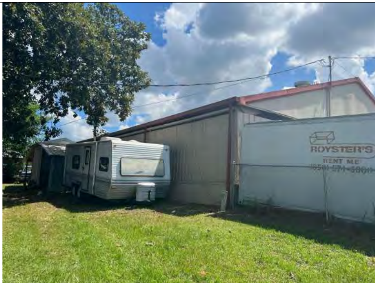
BUILDING 11 PHOTO #5: Partial view of west elevation.
