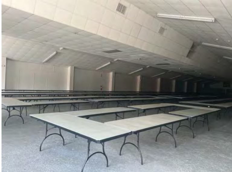
BUILDING 8 PHOTO #25: Interior view of Building 8.
