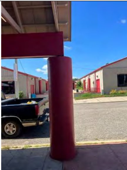
BUILDING C9-C11 PHOTO #7: Concrete column supporting roof overhang at the buildings.
