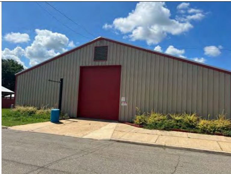
BUILDING 9 PHOTO #1: View of north elevation.
