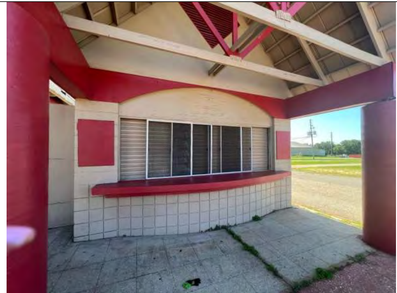
BUILDING C1-C4 PHOTO #8: Typical front elevation of Buildings C1-C4.
