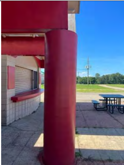
BUILDING C5-C8 PHOTO #7 Concrete column supporting roof overhang at the buildings.
