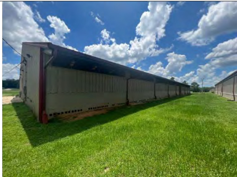
BUILDING 6 PHOTO #3: View of west elevation.
