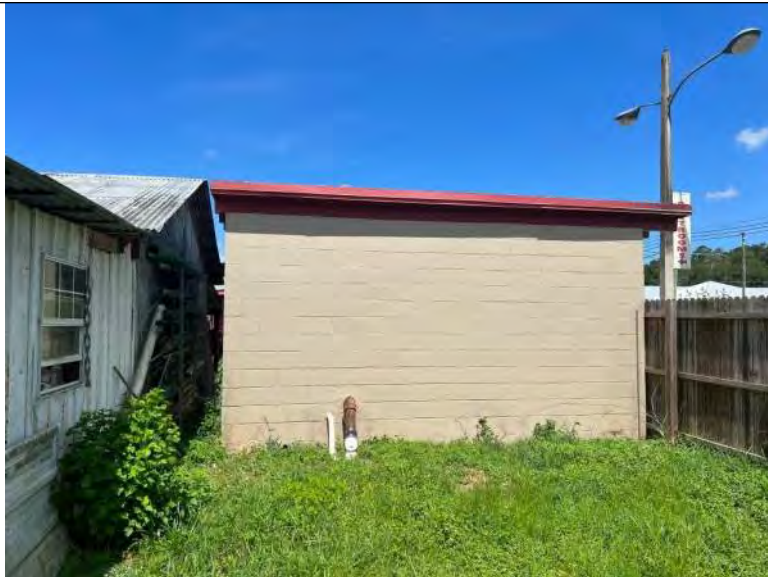
BUILDING R3 PHOTO #5: View of east elevation.
