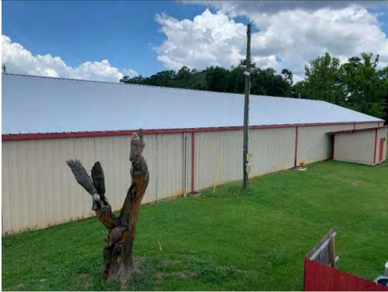
BUILDING 2 PHOTO #13: Overall view of metal roof panels associated with building 2.
