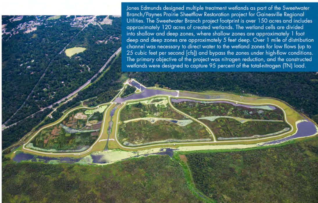
Figure 3 Constructed Wetland Example – Sweetwater Branch
