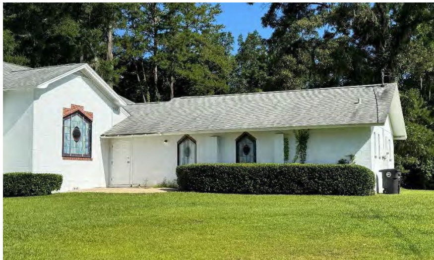
Figure A-5. Concrete block addition at the northeast corner of the east elevation of Testerina Church, facing north.
