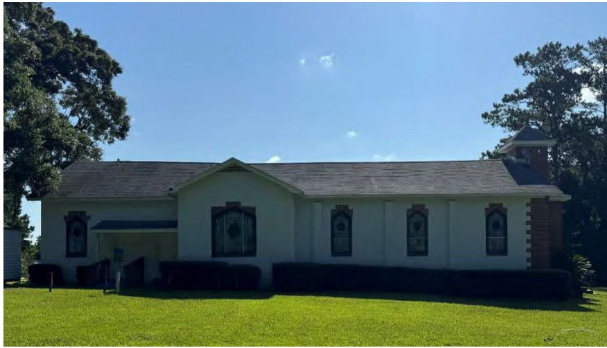
Figure A-3. West elevation of the Testerina Church, facing east.
