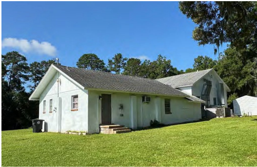
Figure A-4. Concrete block addition at the northeast corner of the east elevation of Testerina Church, facing southwest.
